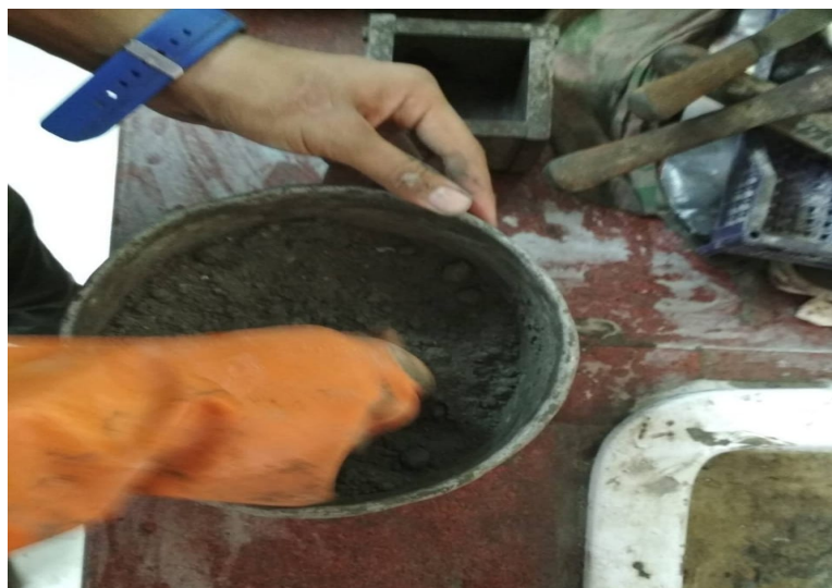
Photo 3.12. Manual Mixing of Grout
