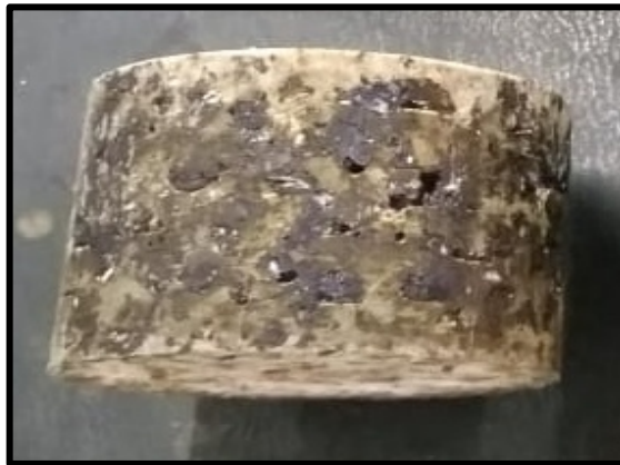
(c) Full depth of grouting
