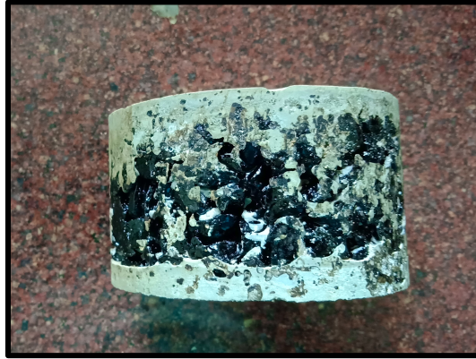
(a) Shallow depth of grouting
