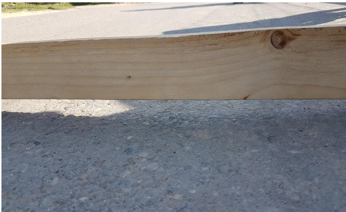
Figure 4.13: Large Rut depth on SN Section
