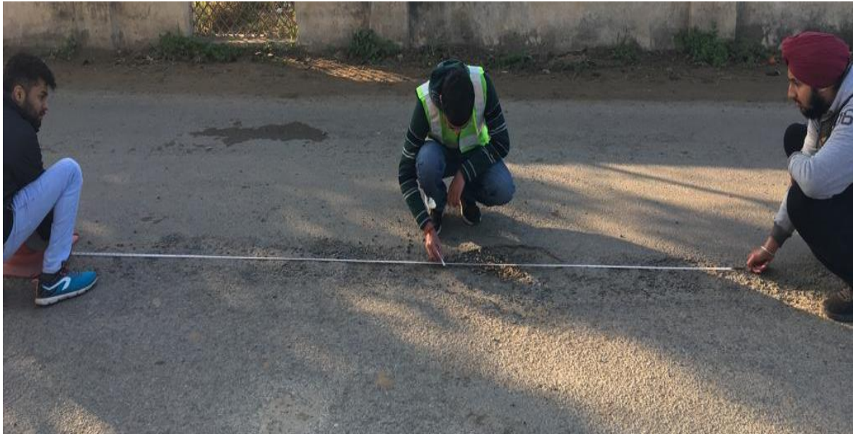
Figure 4.8: Measurement of Ravelling at Section MN
