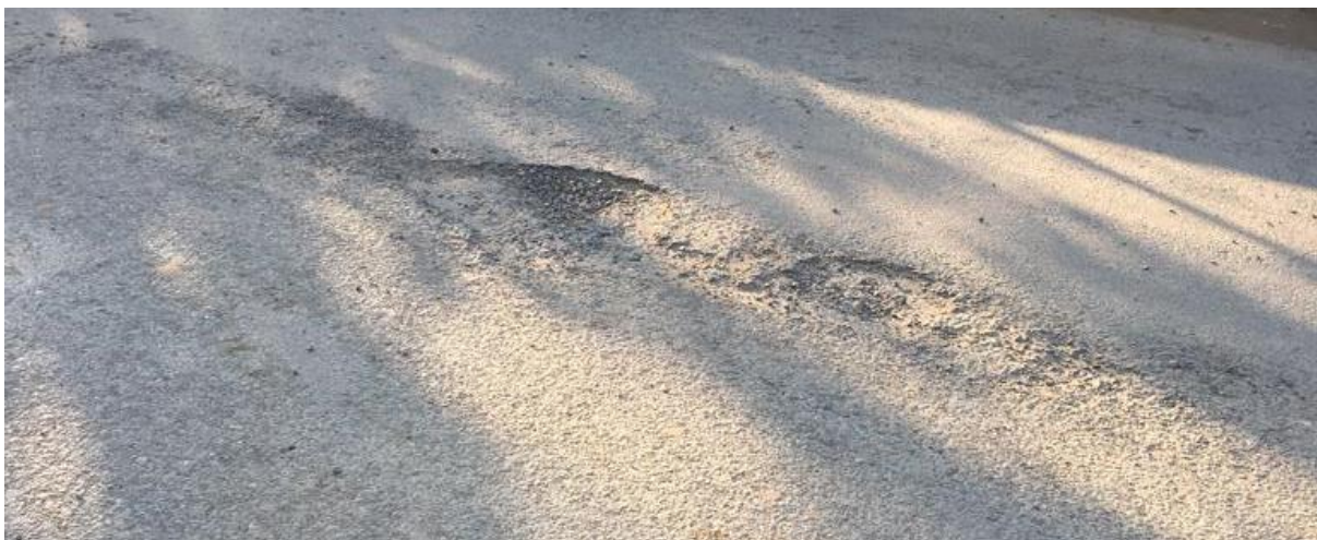
Figure 4.7: Ravelling at Section PN
