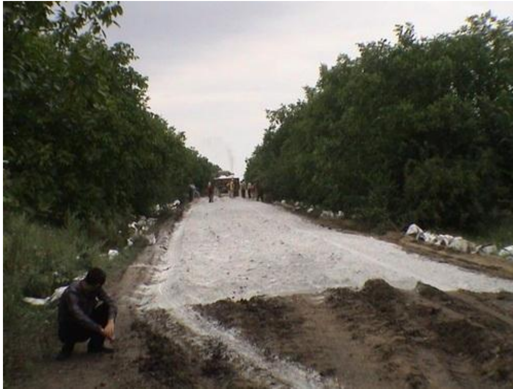
Figure 1.1: Laying of RBI Grade-81 (Source www.rbigrade81.com )
