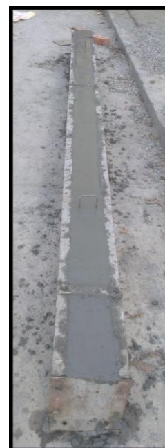
Fig 3.3 Beam after casting
