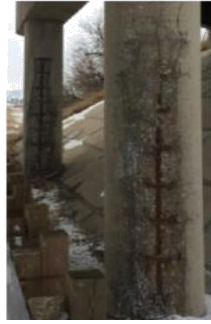
(1) Corrosion in columns
