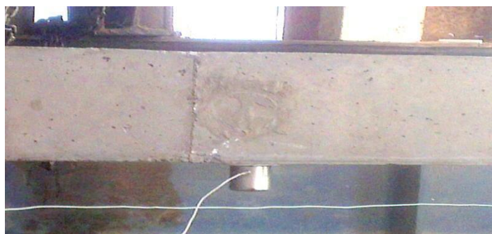
Fig 3.9 Accelerometer placed below at centre position of beam
