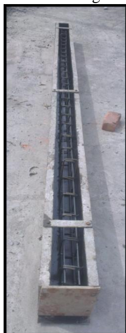
Fig 3.2 Beam mould with reinforcement cage
