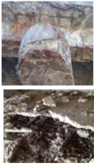
(1) Corrosion in columns
