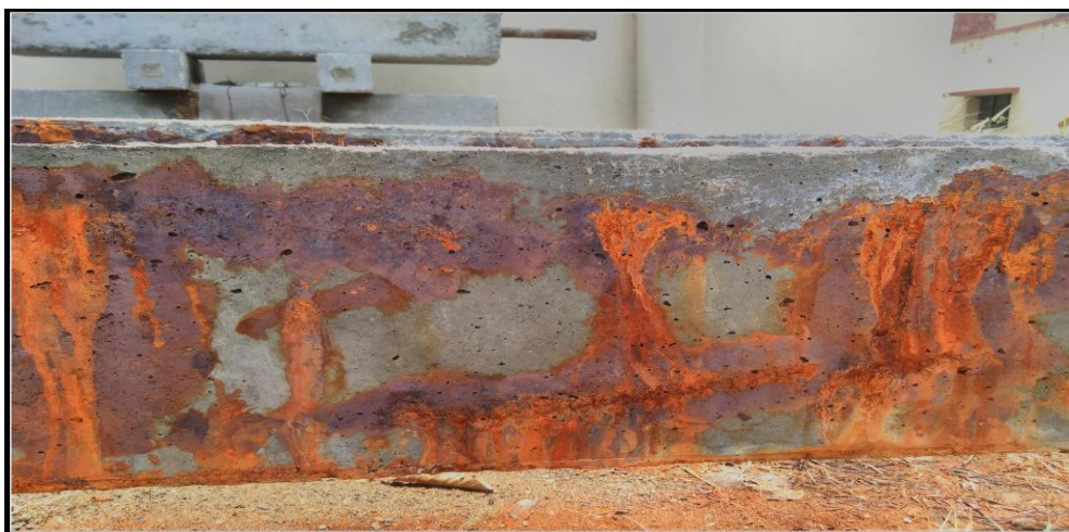
Fig 4. 3 Red brownish products observed along the side
