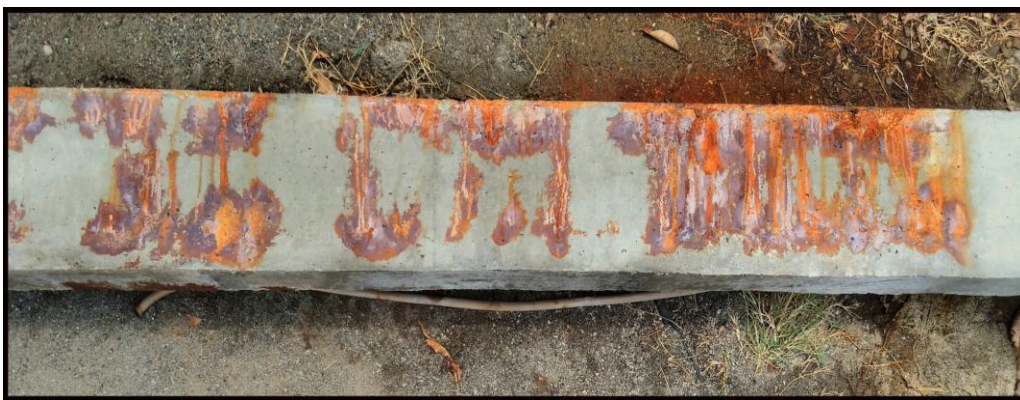
Fig 4.2 Right side of front face of C-7
