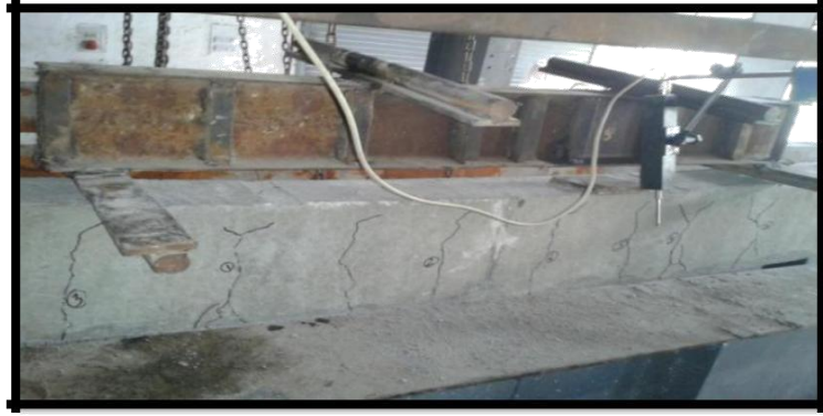
Fig 4.13 Flexure Cracks on side face of C-0 beam
