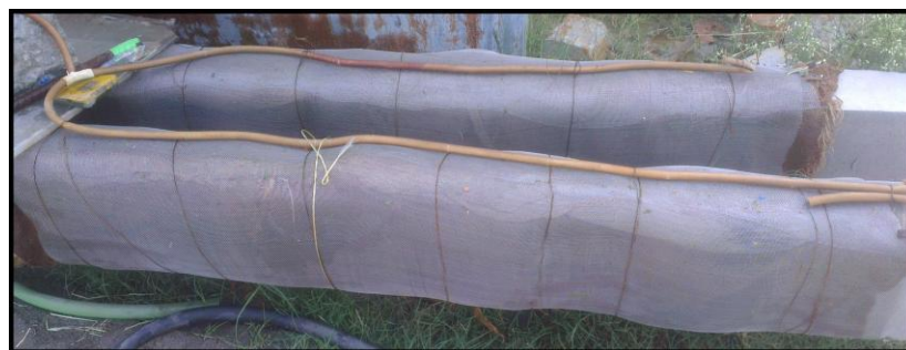
Fig 3.5 Stainless steel wire mesh wrapped around central 1.5 m part of Concrete beam served as cathode
