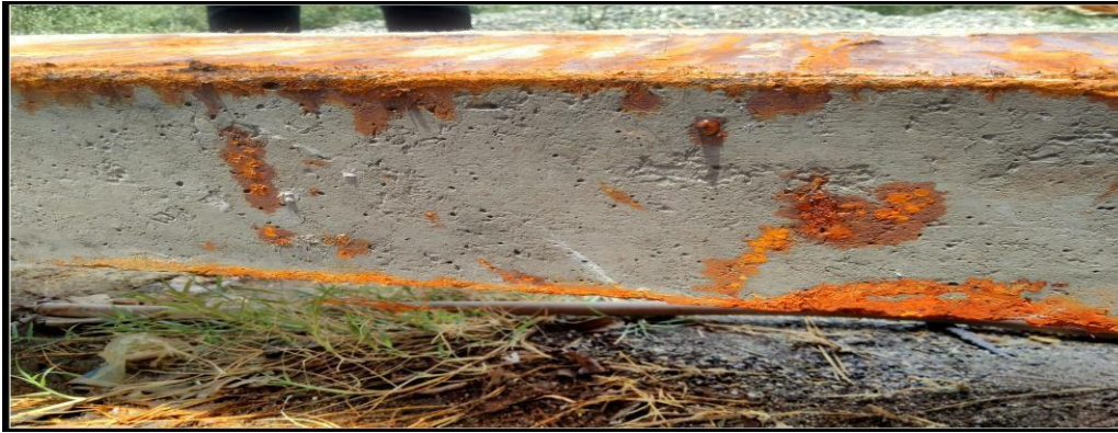
Fig 4.1 Bottom face of C-7
