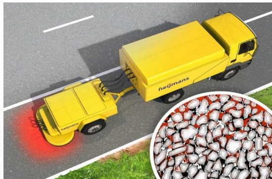
Figure 20 Self-Healing of Asphalt Pavement by IR Induction
