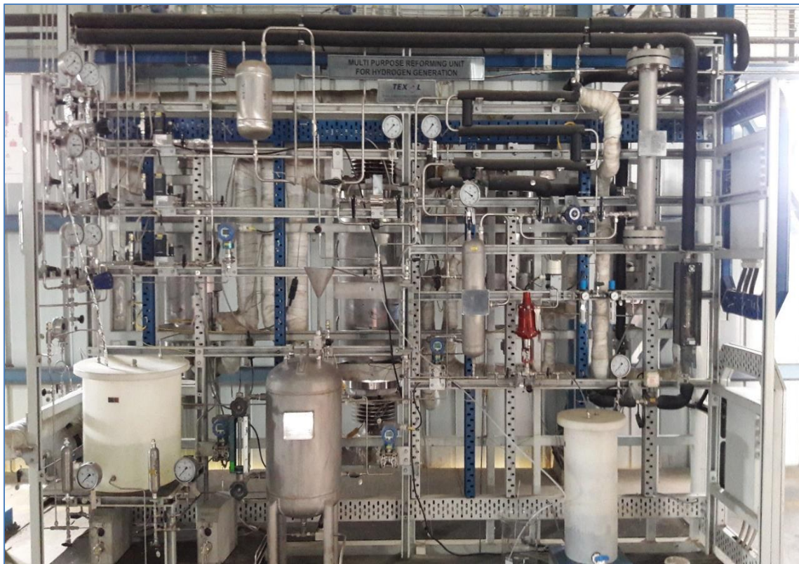
Figure 29 Multi-Purpose Reforming Unit
