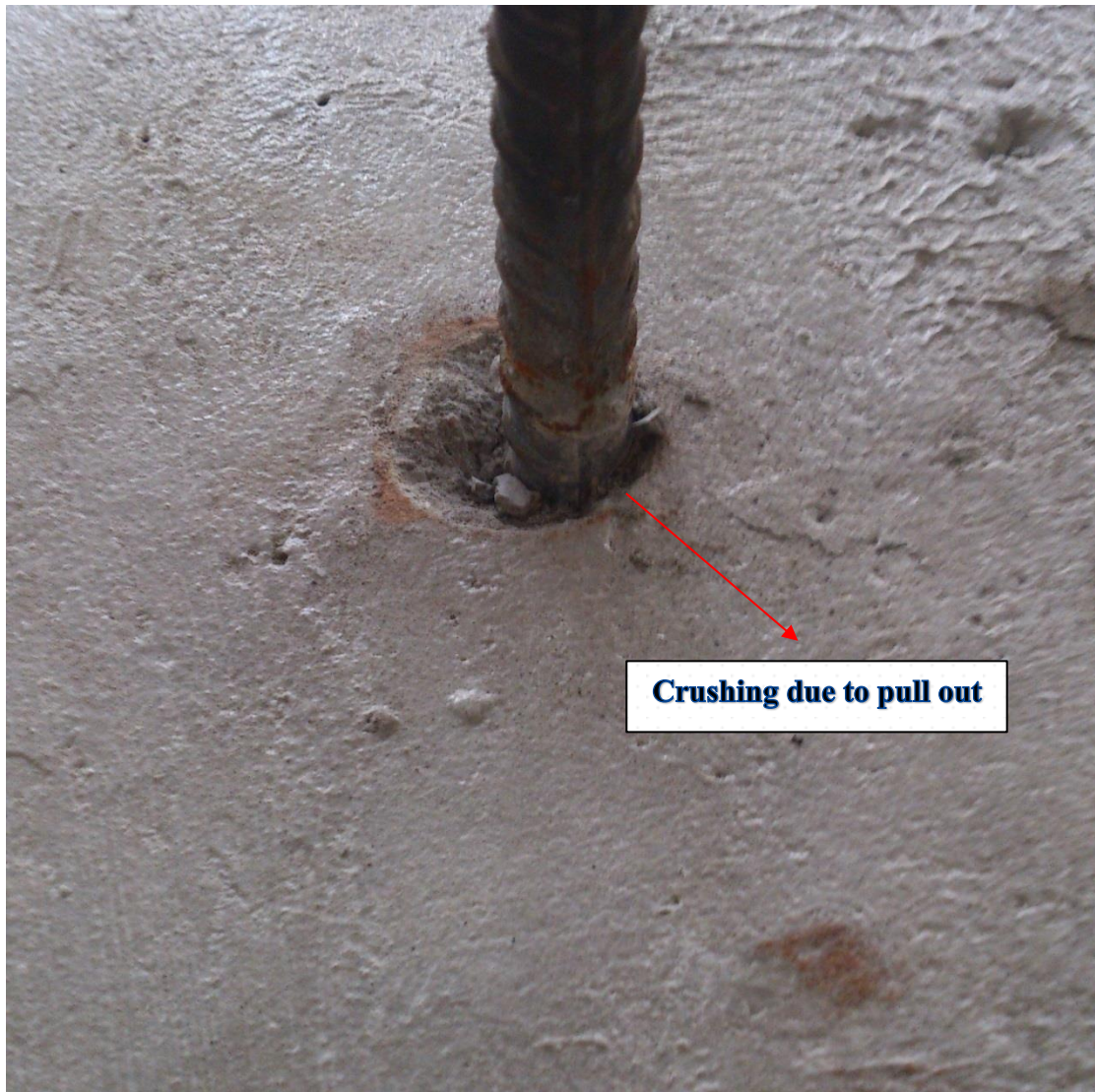
Figure 3.11: Crushing due To Pull out Bar Lugs after Pull out Test
