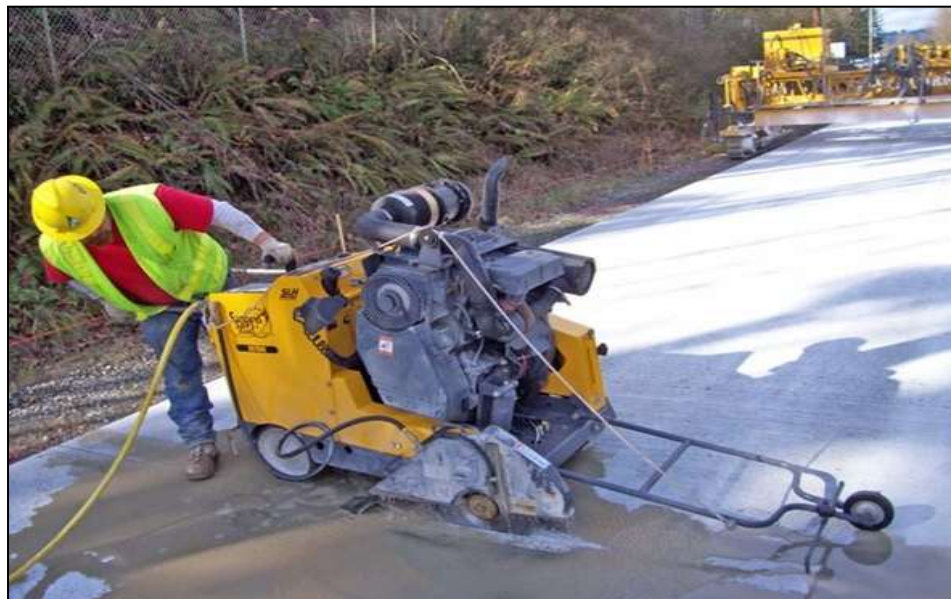
Fig. 1.11 Saw cut in transverse direction
