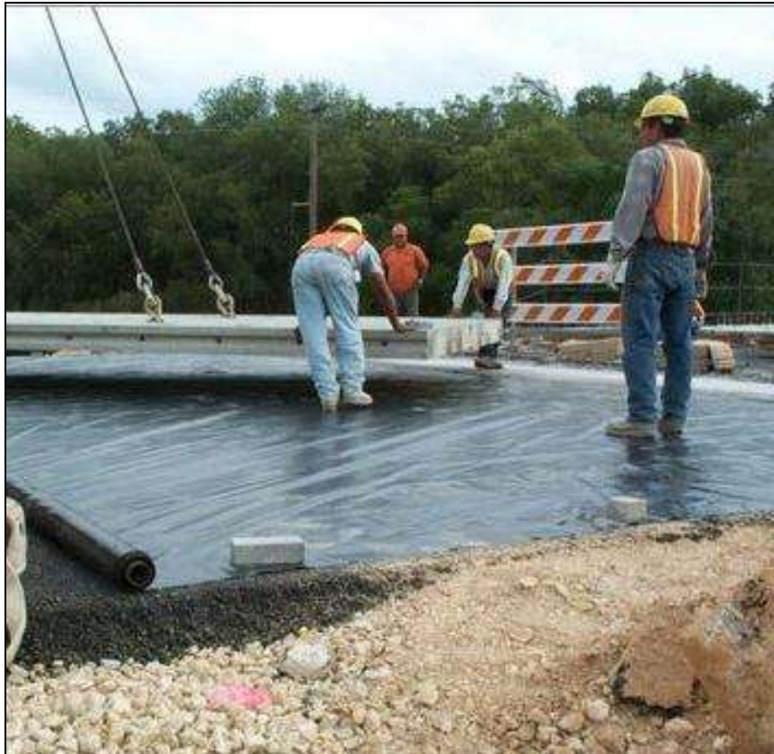
Fig. 1.9 Laying of separation membrane
