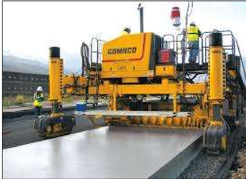
Fig. 1.16 Laying of Pavement Quality Concrete (PQC) with Slip Form Paver
