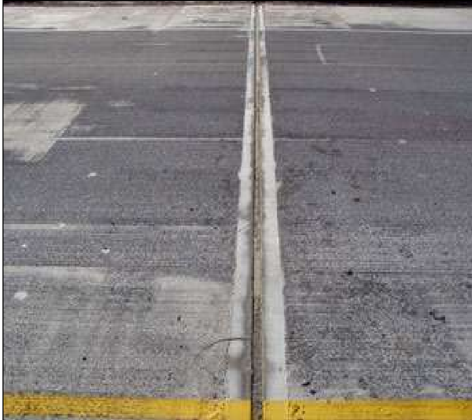
Fig. 1.10 Longitudinal joint in Pavement Quality Concrete (PQC)
