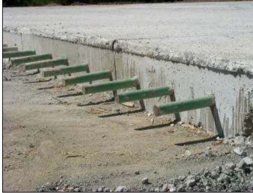
Fig. 1.14 Dowel bars in Pavement Quality Concrete (PQC)
