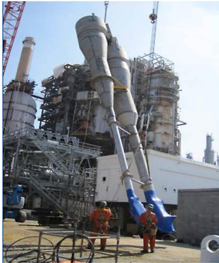
Fig. 4: A typical two-stage cyclone system (Sadeghbeigi, 2012).
