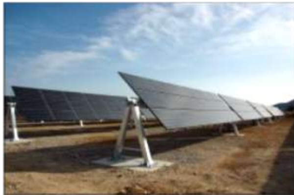
Figure 1.5 A single axis horizontal tracking system [Cheema, S S 2012]
