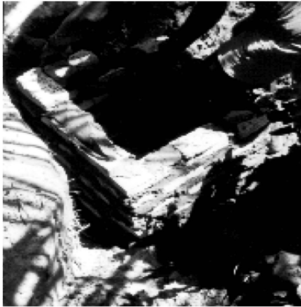
Fig: 2.2 Simplified brick junction chamber
