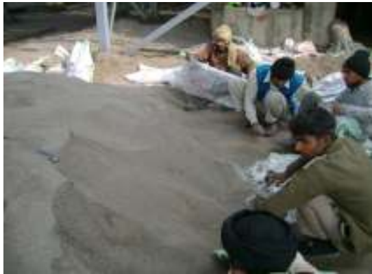
Figure 5.6 Labourers cleaning sand at JPP
