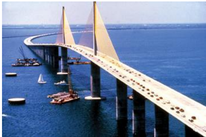
Figure 2.3: Fly ash concrete used in severe exposure applications ( https://www.fhwa.dot.gov )
