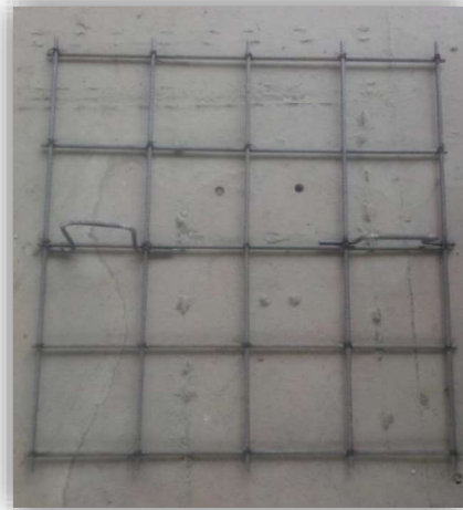
Fig. 4.5: R/F of 190 mm spacing
