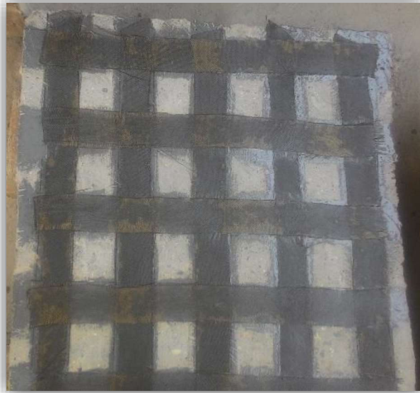
Fig. 5.1: Strengthening of slab using BFRP
