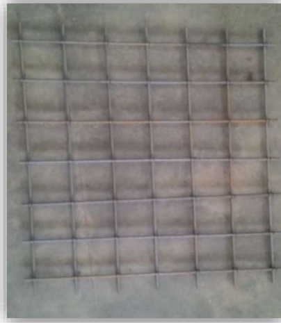
Fig. 4.3: R/F of 120 mm spacing
