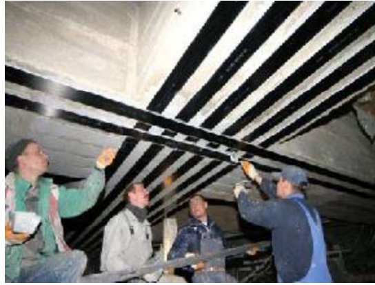
Fig. 1.8: Flexural strengthening of concrete girder
