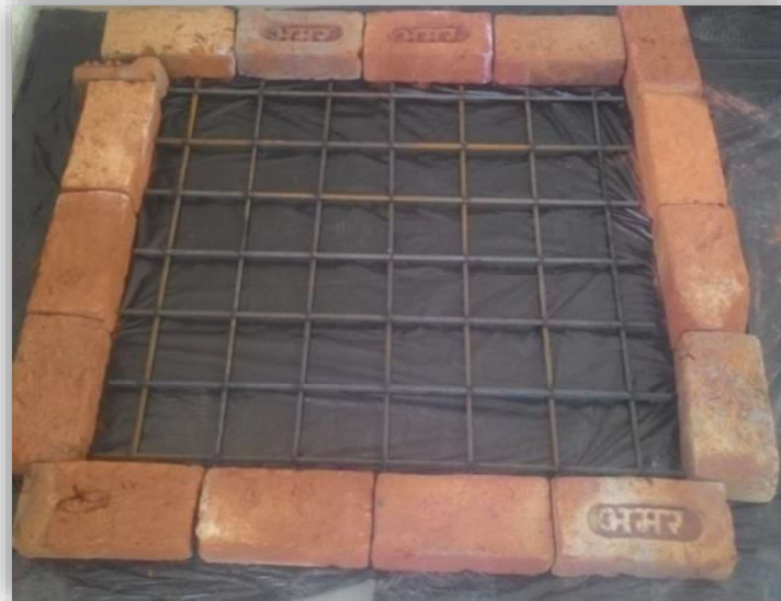
Fig. 4.1: Slab casting formwork
