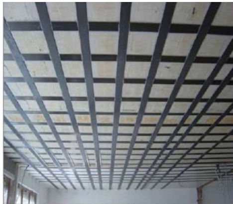
Fig. 1.9: Strengthening of a concrete deck using CFRP strips
