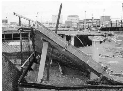
Fig. 1.10: Punching shear failure (stucturemag.org)
