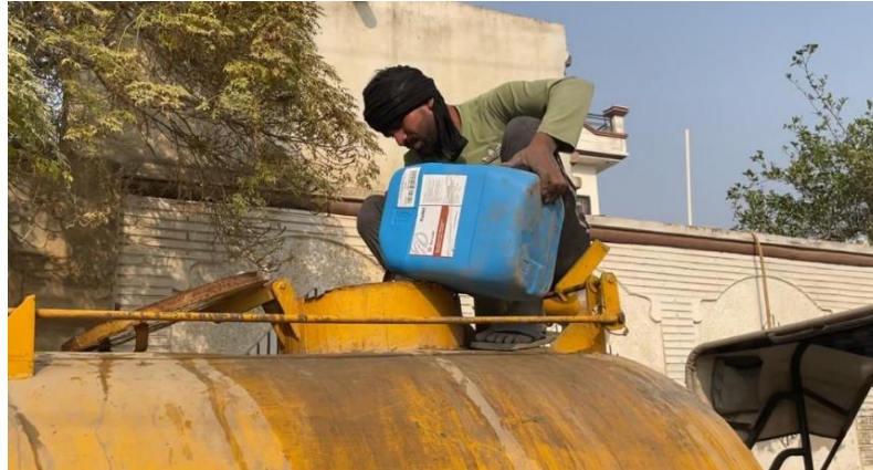
Figure 4.8: Mixing Chemical (Terracil and Zycobond)
