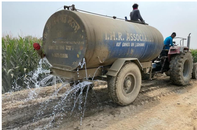
Figure 4.9: Spreading Chemical (Terracil and Zycobond) on Sections.
