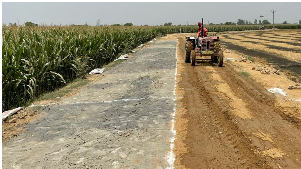
Figure 4.5: Spreading of Cement on different sections
