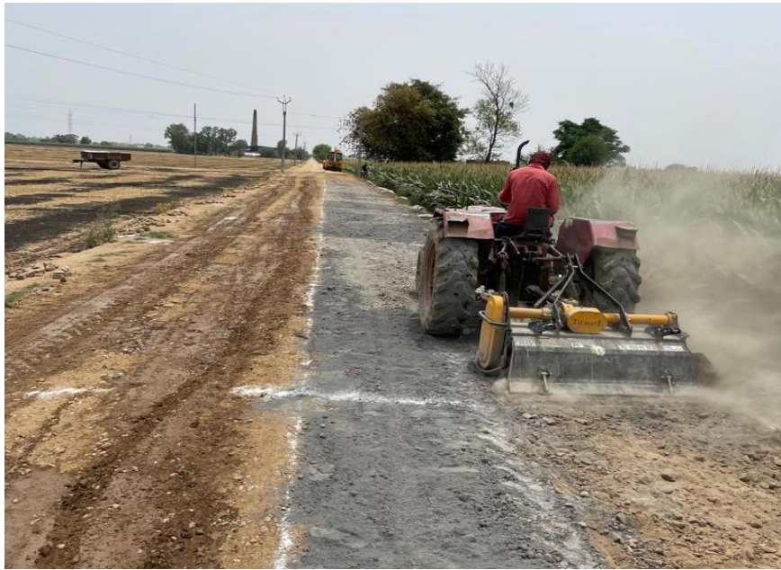
Figure 4.6 : A Rotavator: Blending of cement, soil and aggregates.
