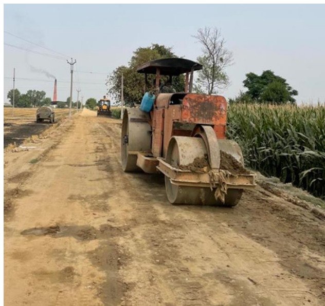
Figure 4.11: Compaction using 3 drum roller
