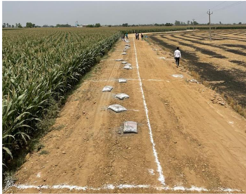
Figure 4.4: Marked area for spreading of cement.
