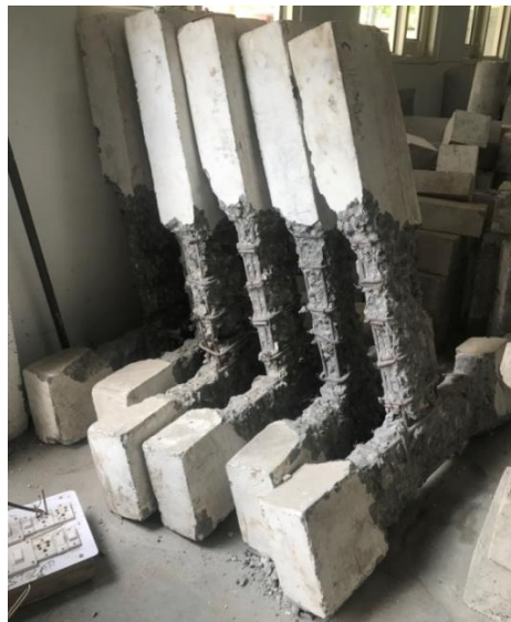
Fig. 4.14 - Specimen Chipped Off for the Retrofitting
