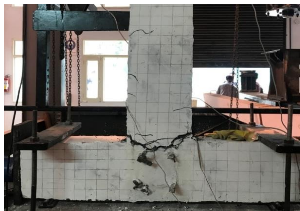
Fig. 5.33 - Failure of R-CD at Ultimate Lateral Displacement (Specimen 2)
