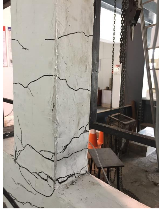
Fig. 6.7 - Side View of the Crack Pattern of Control Severe Damage (CSED) Specimen I
