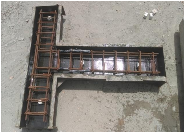
Fig. 4.7 – BCJ Reinforcement Cage is Placed Inside of the Mould
