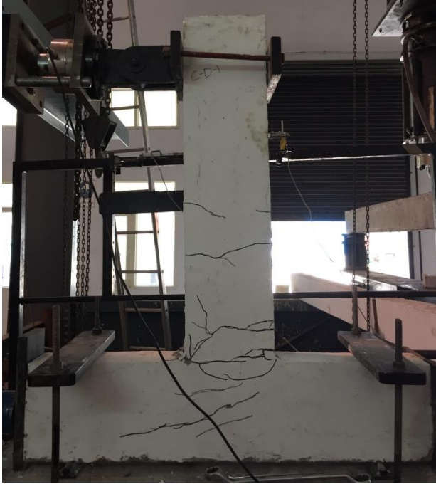
Fig. 6.6 - Crack Pattern of Control Severe Damage (CSED) Specimen I
