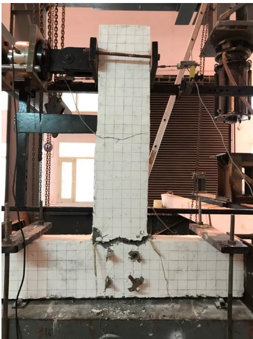
Fig. 6.35 - Crack Pattern of Wire Mesh Confined HP-HFRC Retrofitted Control Damage (WC-RCD) Specimen II
