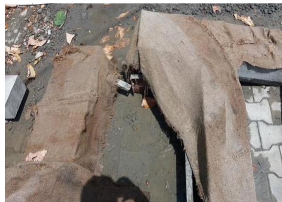
Fig. 4.10 - BCJ Surface Cover with Wet Jute Bags for Curing
