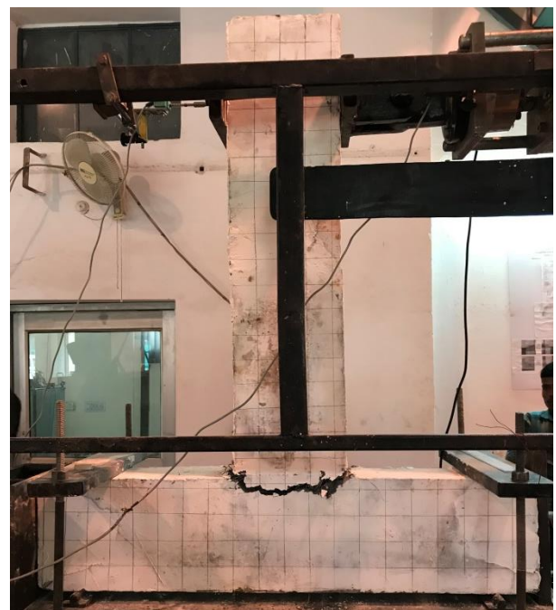
Fig. 6.36 - Back View of the Crack Pattern of Wire Mesh Confined HP-HFRC Retrofitted Control Damage (WC-RCD) Specimen II
