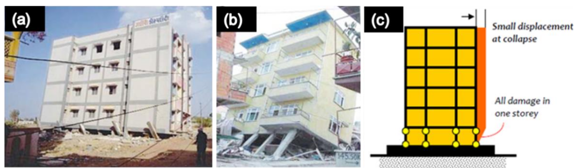
Fig. 1.5 – (a) Building Collapse Due to Soft Story During the Gujarat Earthquake M 7.7 (Patnala et al., 2016), (b) Soft Story Failure Observed During Earthquake in Turkey M7.4 (Patnala et al., 2016) (c) Schematic Representation of Damage Location in Soft Story Failure (Murthy et al., 2012)
