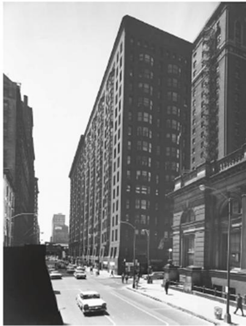
Fig. 1.2 - Tallest Load-Bearing Brick Structure in the World “Monadnock Building, 1889” Stored in Chicago Historical Society (HB-19320-C). (Photographer: Hedrich Blessing.)
