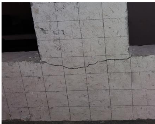
Fig. 5.11 - Crack Pattern of Control Slight Damage (C-SD) Specimen I
