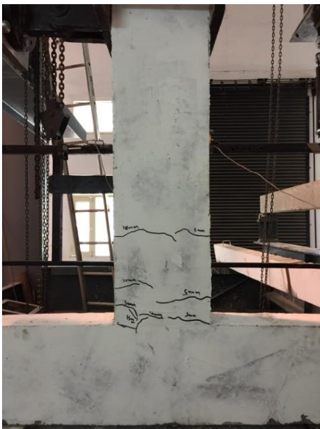
Fig. 6.10 - Crack Pattern of Control Moderate Damage (CMD) Specimen I
