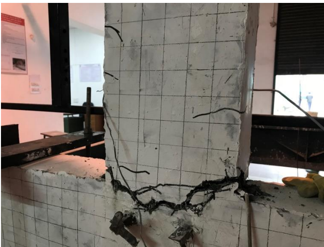
Fig. 6.39 - Crack Pattern of Wire Mesh Confined HP-HFRC Retrofitted Severe Damage (WC-RSED) Specimen II
