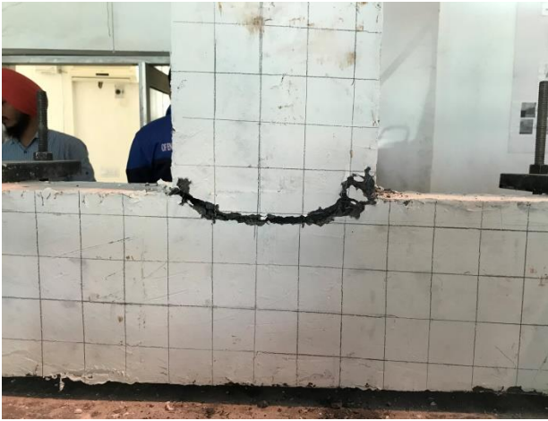
Fig. 6.41 - Crack Pattern of Wire Mesh Confined HP-HFRC Retrofitted Moderate Damage (WC-MD) Specimen I
