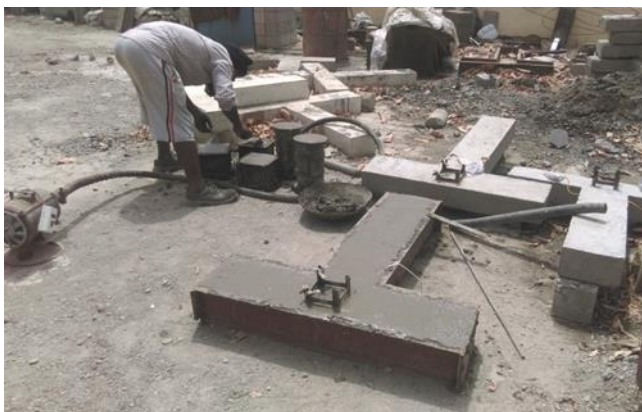
Fig. 4.9 - Cubes and Cylinders Filled for 28 Days Compressive Strength Testing
