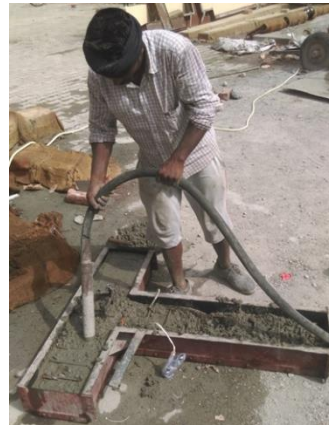
Fig. 4.8 - Internal Type Vibrator used for Compaction
