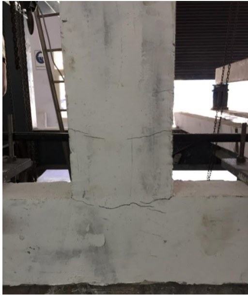
Fig. 6.15 - Crack Pattern of Control Slight Damage (CSD) Specimen I
