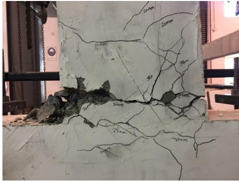
Fig. 6.4 - Crack Pattern at 25 mm Lateral Displacement of Control Severe Damage (CCD) Specimen II
