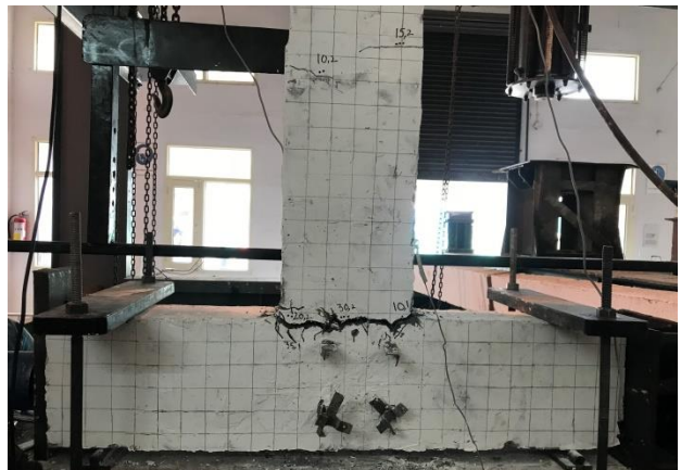
Fig. 5.39 - Failure Pattern of R-SD at Ultimate Lateral Displacement (Specimen 2)
