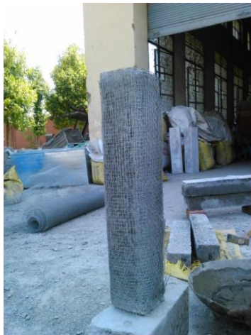
(c) Three layer GI Wire Mesh Jacketing
