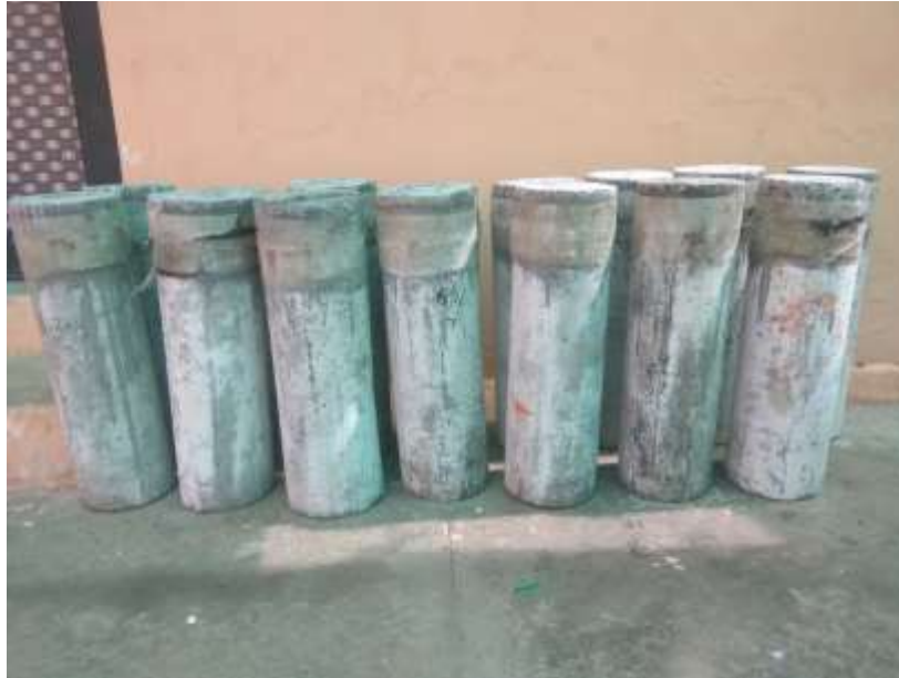
Figure 3.10 GFRP wrapped at top of columns
