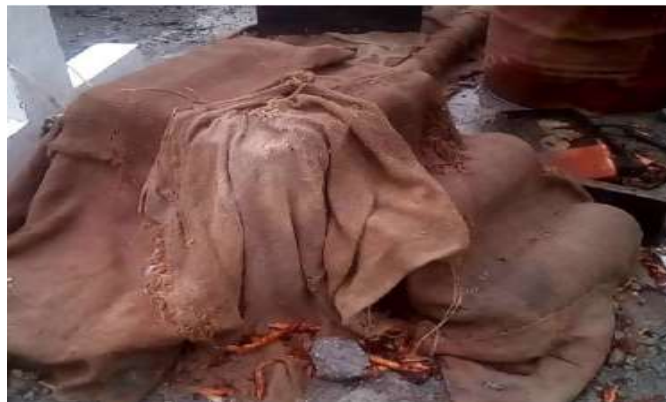
Figure 3.9 Curing of column specimen using jute sacks
