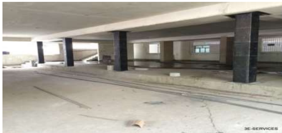
Figure 1.8 Columns wrapped with FRP externally ( http://www.3eservices.net )
