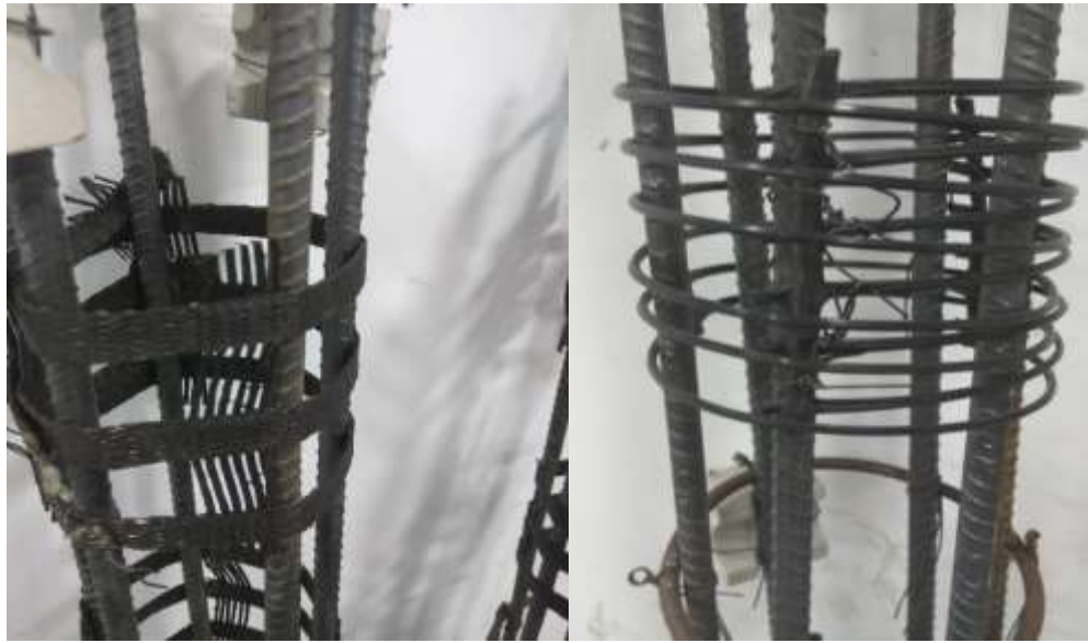
Figure 3.6 Application of geo-grids
