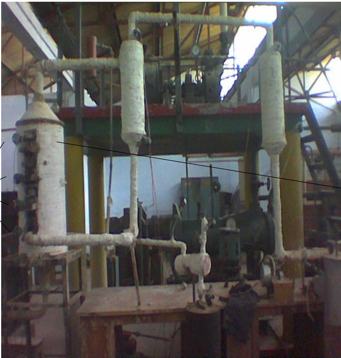
Fig. 5.2: Furnace with firing windows
