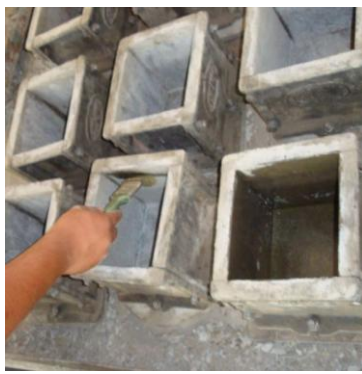
e) Oiling of mould
