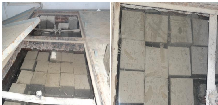
b) Curing of concrete in water tank
