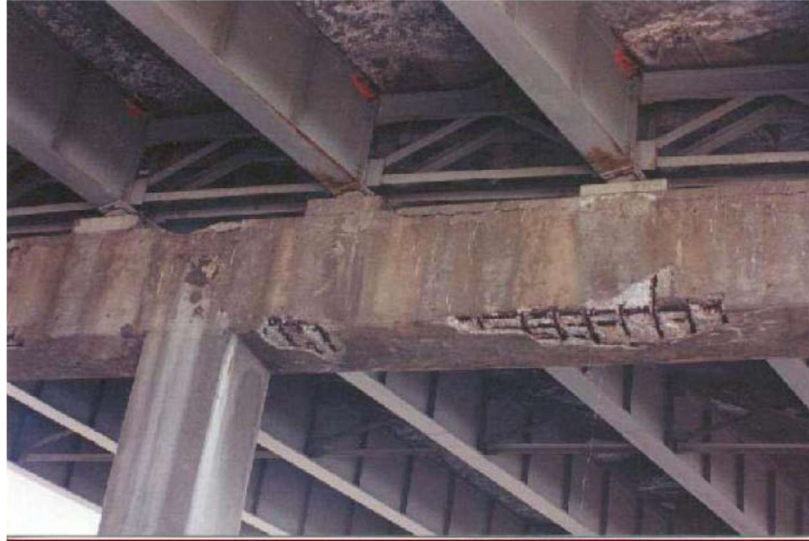
Figure 1.1 Corrosion of a cross girder that supports the main bridge deck ( www.concretebridgesview.com )
