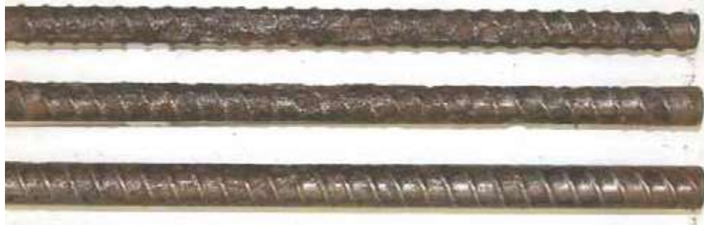
Figure 1.11 Pitting corrosion on Steel rebars.
