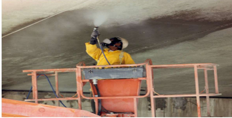
Figure 2.1 Application of surface inhibitor ( http://www.tecnoconverting.com )
