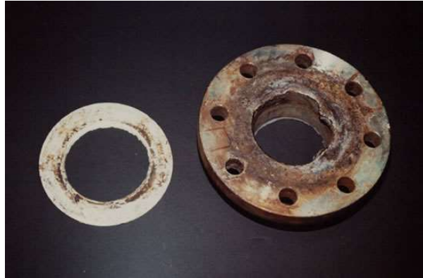
Figure 1.9 Crevice corrosion on a stainless steel flange exposed to a chloride-rich medium. ( http://www.cdcorrosion.com )
