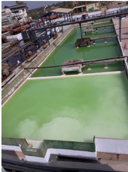
Fig. 14: Treated Effluent Holding Tank of CETP
