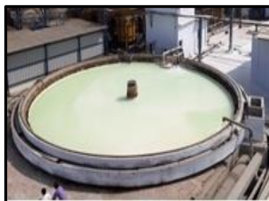
Intermediate holding tank
