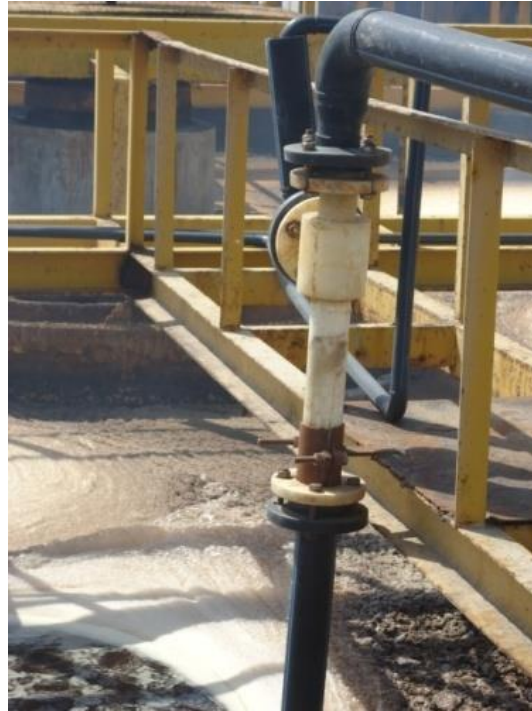
Fig. 8: Hydrodynamic Cavitation Reactor
