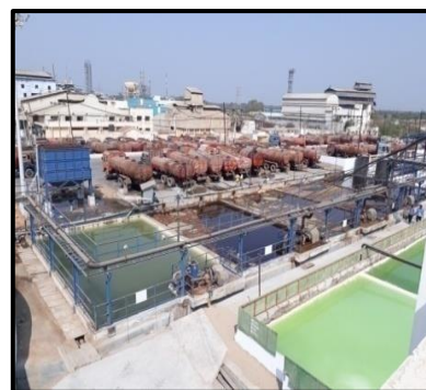
5 Collection tanks in the middle of tankers and mixing tank
