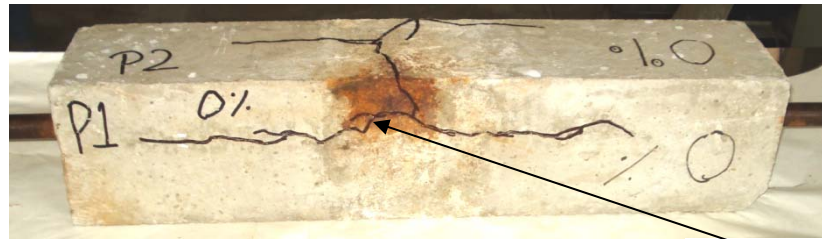
Localized & Small corrosion product
