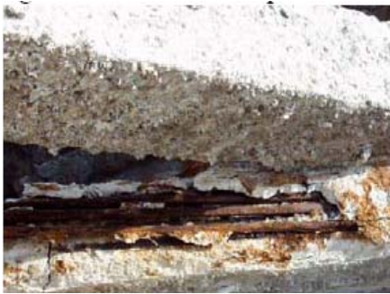
Fig. 3.16: Critical Stages of corrosion in main beams of a dock structure
