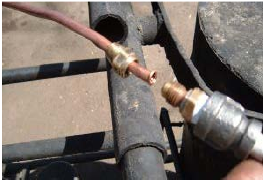
Figure 3.19 - Flared connections [32]
