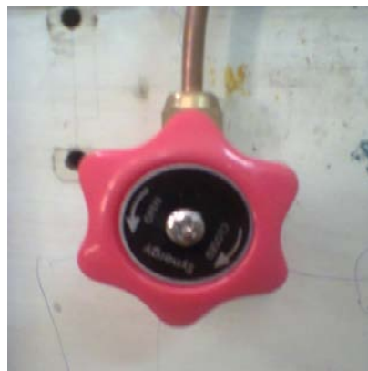
Figure 3.17 - Hand shut valve
