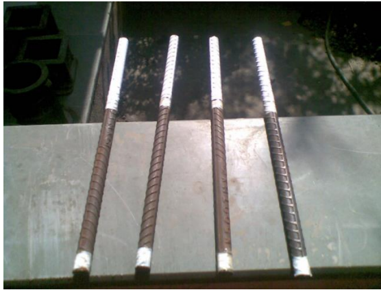
Fig. 3.3. Steel reinforcing bars before casting
