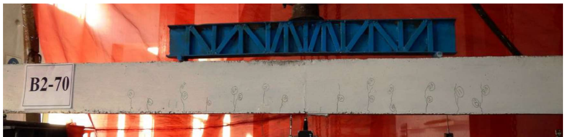
Fig.4. 5 Crack patterns of beam B2-70 when specimen was loaded upto 7kN.
