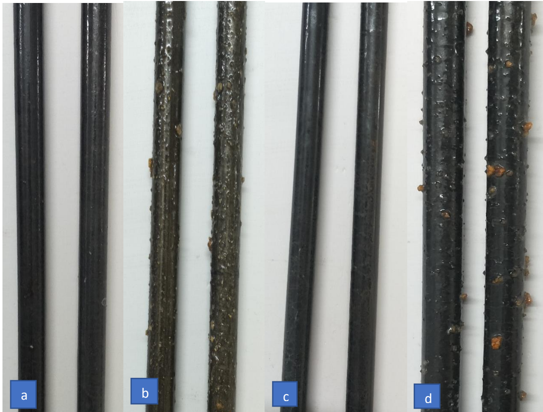
Figure 3.11: Coated rebar; (a) PC, (b) MC, (c) NC, (d) MNC.
