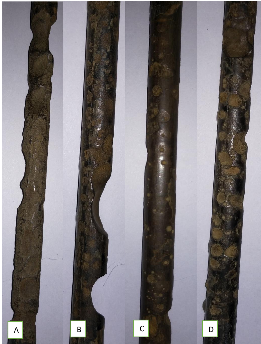
Figure 4.26: Corroded plain mild steel rebar, (A) PC rebar after 18 days, (B) NC rebar after 41 days, (C) MC rebar after 60 days, (D) MNC rebar after 60days of corrosion.
