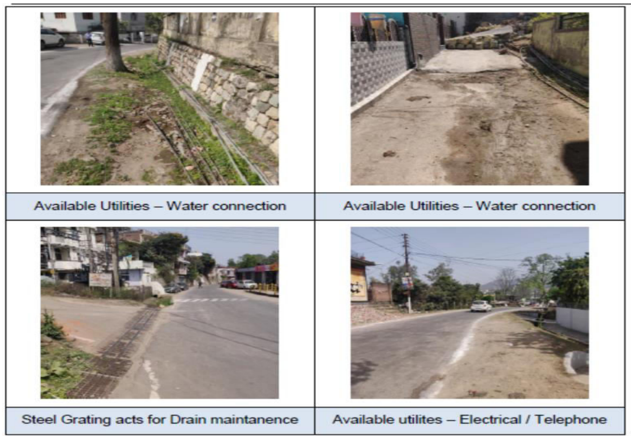
Fig.3.12: Road Inventory Photographs
