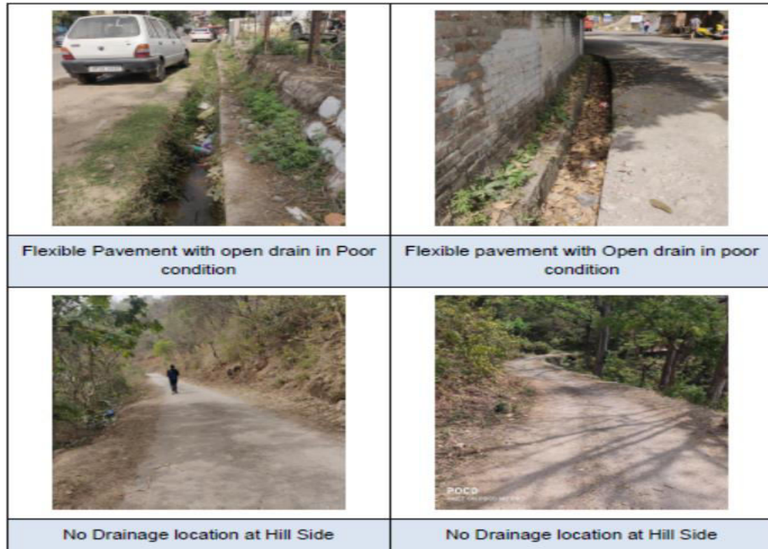
Fig.3.14: Drain Inventory Photographs
