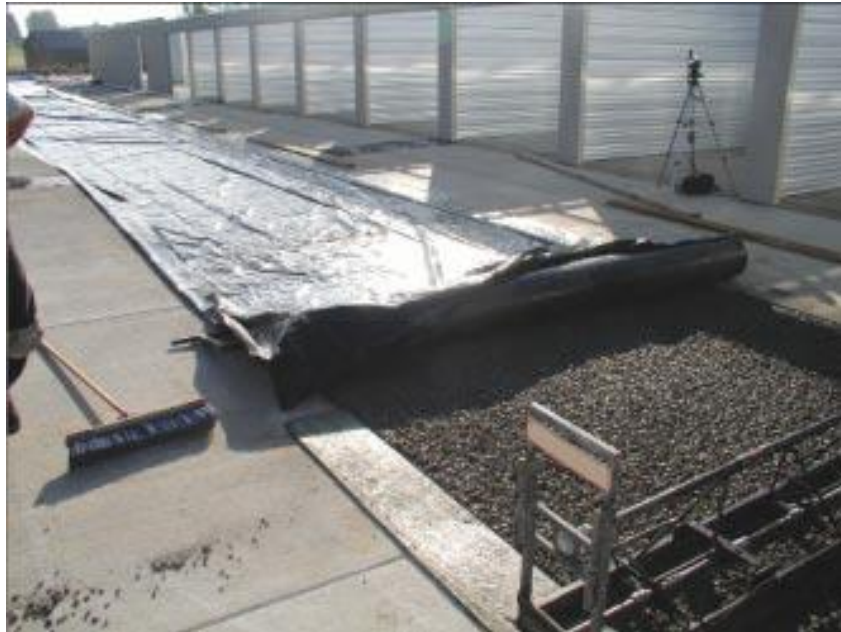
Figure 1.6: Plastic sheeting to cover Pervious Concrete (Image Source: Tennis et al. 2004)
