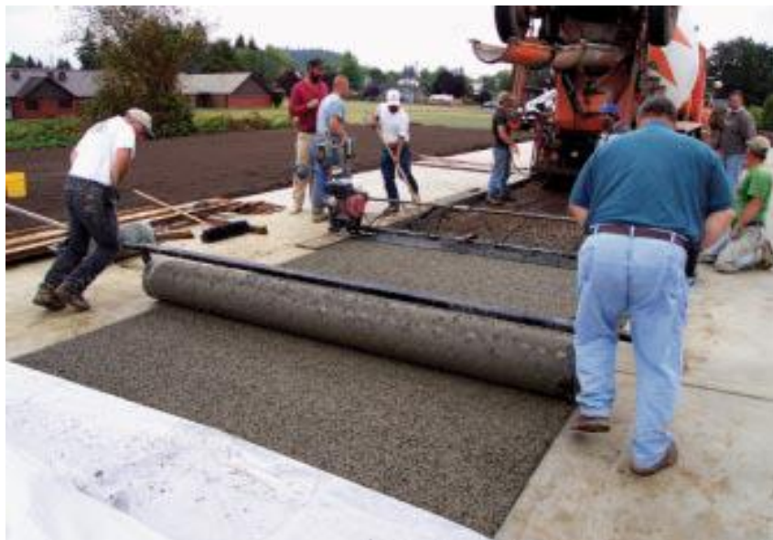
Figure 1.3: Compaction by steel roller (Image Source: Tennis et al. 2004)
