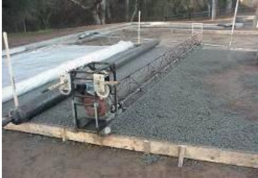
Figure 1.4: Compaction by longitudinal roller (Image Source: Tennis et al. 2004)
