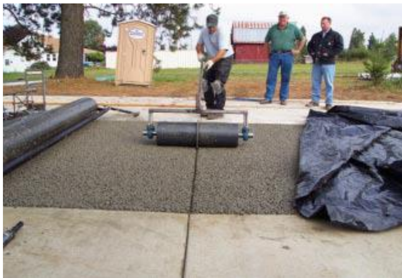
Figure 1.5: Roller joint tool (Image Source: Tennis et al. 2004)
