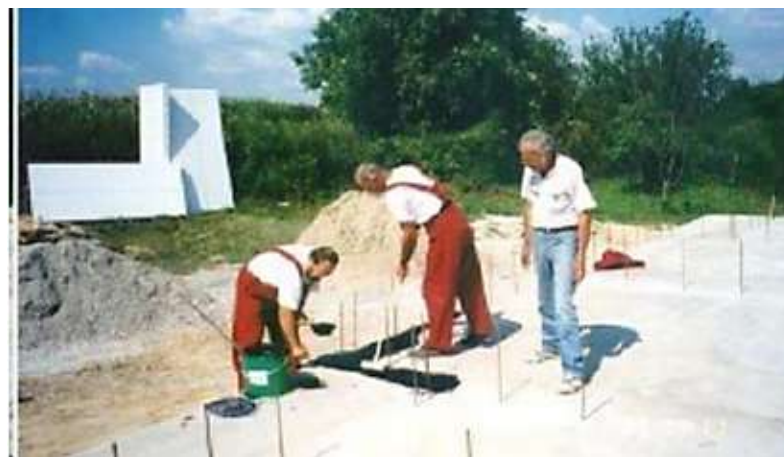
Figure. A 1.1: Groundwork of foundation (EVG)
