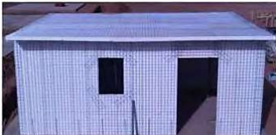
Figure. A.1.10: Roof board setting (BMTPC)
