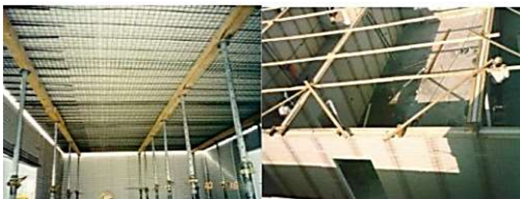
Figure A 1.4. Prop supported for slab construction (EVG)
