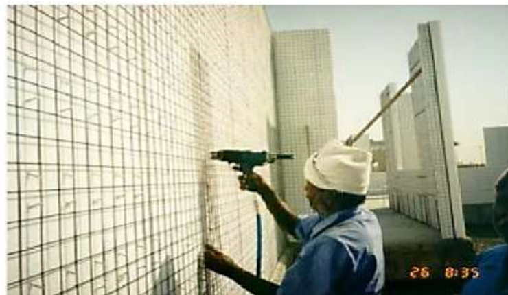
Figure A 1.3. Erection of 3D Boards (EVG)
