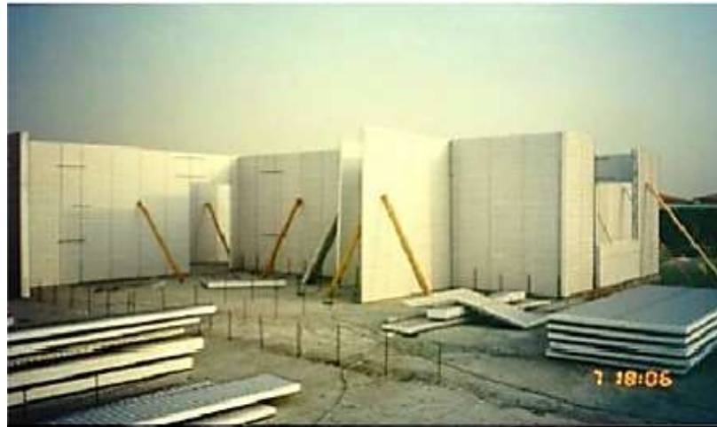
Figure A 1.2. Placement of 3D wall boards for construction (EVG)
