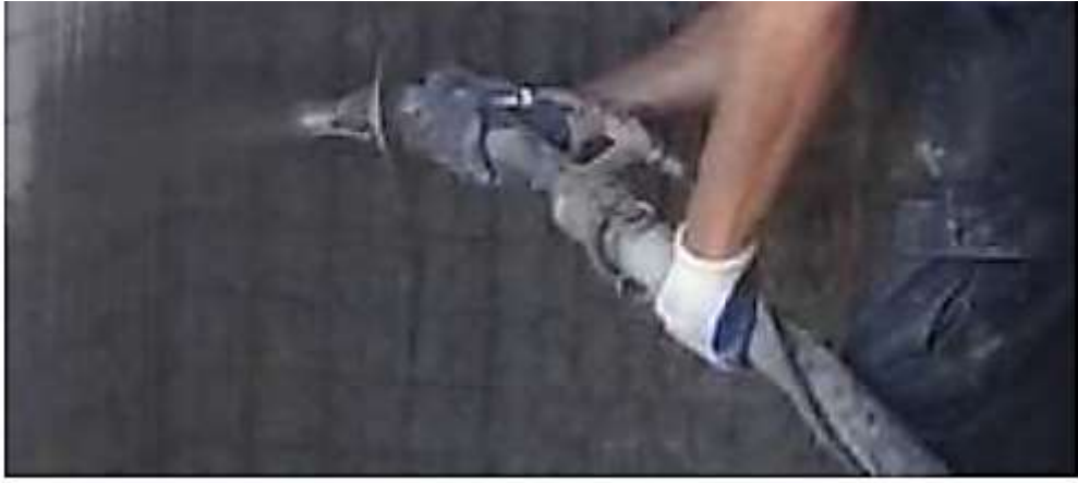
Figure. A.1.11: Process of shotcreting (BMTPC)
