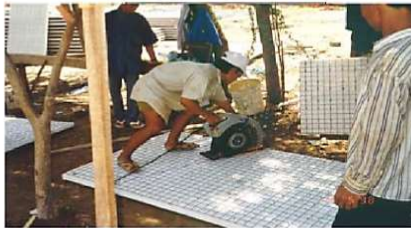
Figure A.1.5. 3D Board cutting method (EVG)
