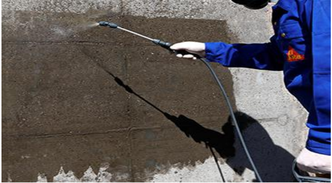
Figure 1.6: Spraying of Corrosion Inhibitors
