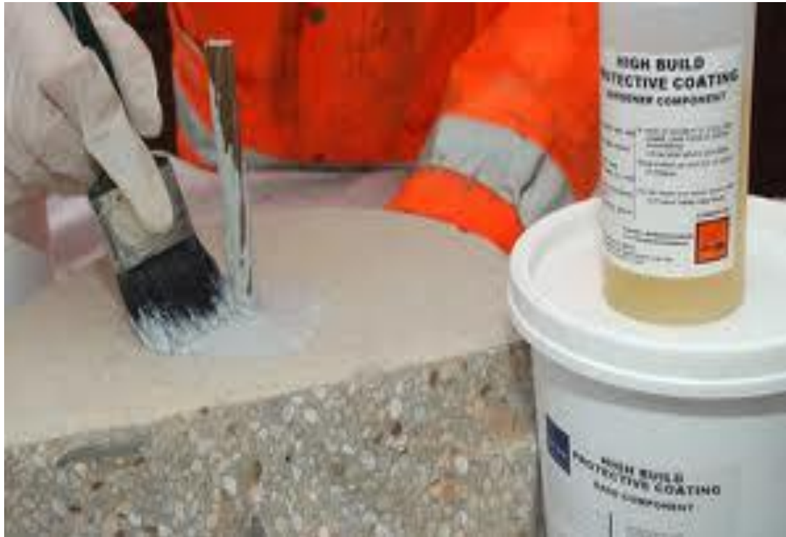
Figure 1.5: Surface Application of Corrosion Inhibitor
