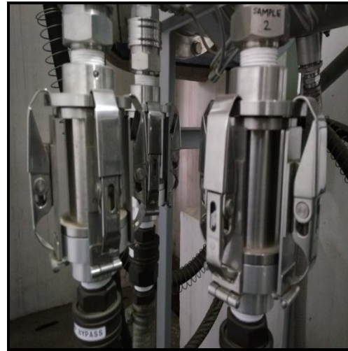
Figure 4.12 Main line filter holder
