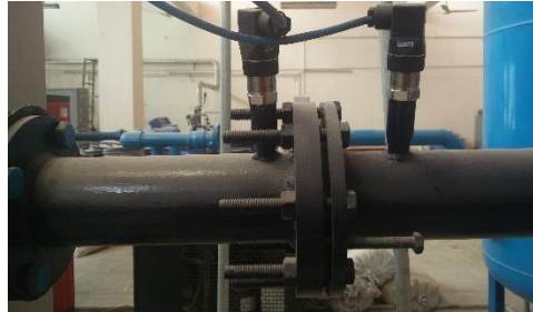
Figure 2.12 : Bolt arrangement for 3-inch flowmeter
