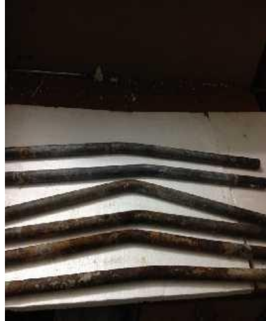
Fig.5.11 Corroded Bars of 25 mm dia
