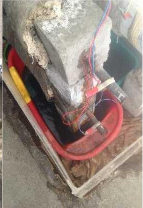
Fig.4.5 Electrical connection to the steel
