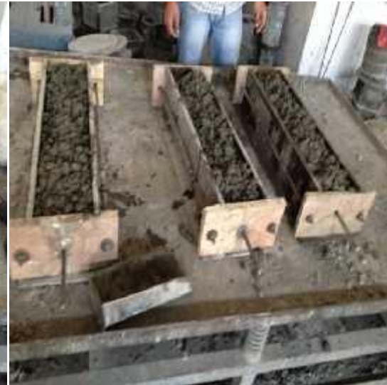
Fig.4.3 Pouring of concrete mix placed on vibrator.
