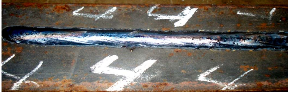
Figure 3.3: Work Plate after Welding
