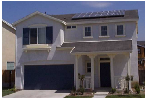
Figure 13: Roof Mount PV System
