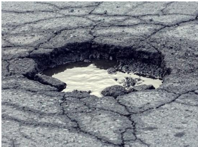
Plate 1.4 Formation of Pothole
