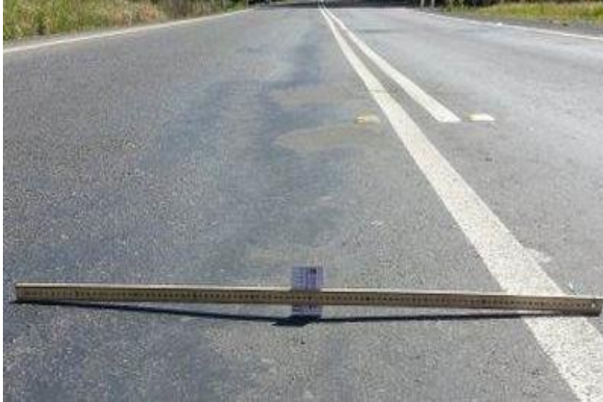
Plate 1.3 Rutting Failure
