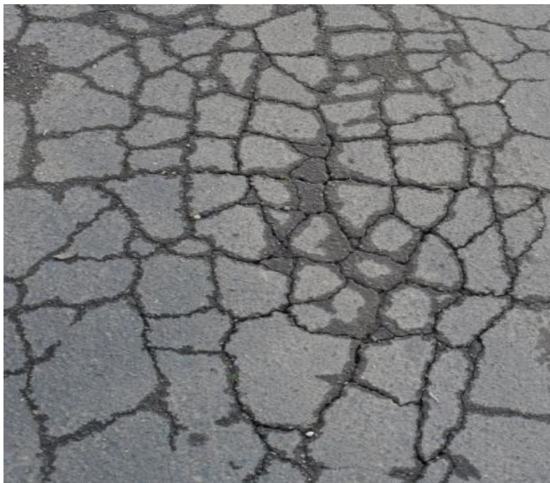
Plate 1.2 Fatigue Cracking
