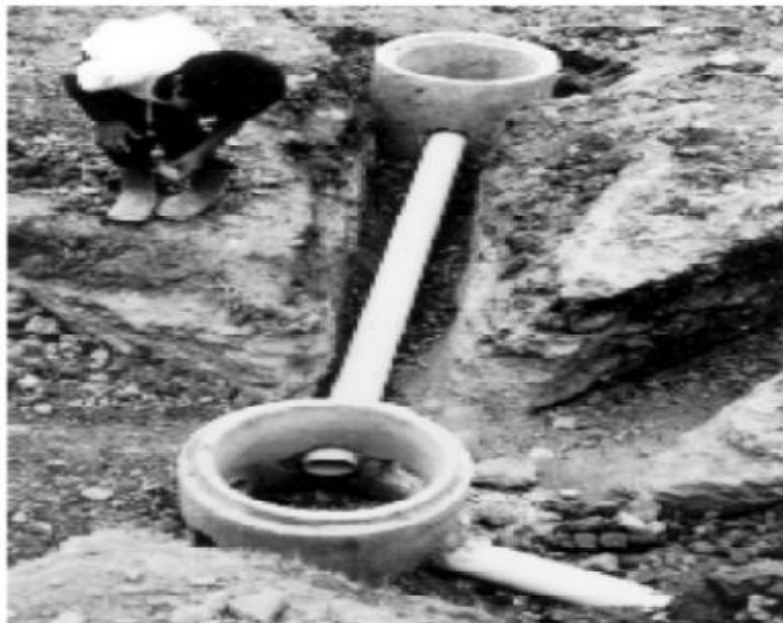
Figure 1.6 Precast Concrete Inspection Chamber (Source: Mara D, Sleigh , 2001)
