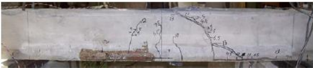
Fig. 3.10 Crack pattern in beam with FRP form and sand aggregate bonded (Bank et al., 2010)
