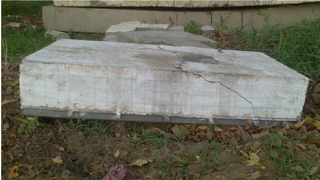
Fig 6.4 shear crack in specimen 2
