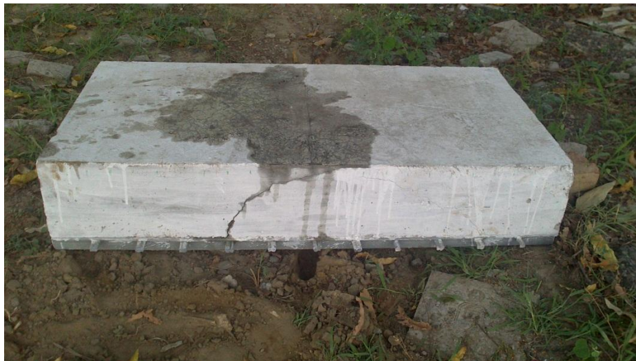
Fig 6.5 cracks in specimen 3
