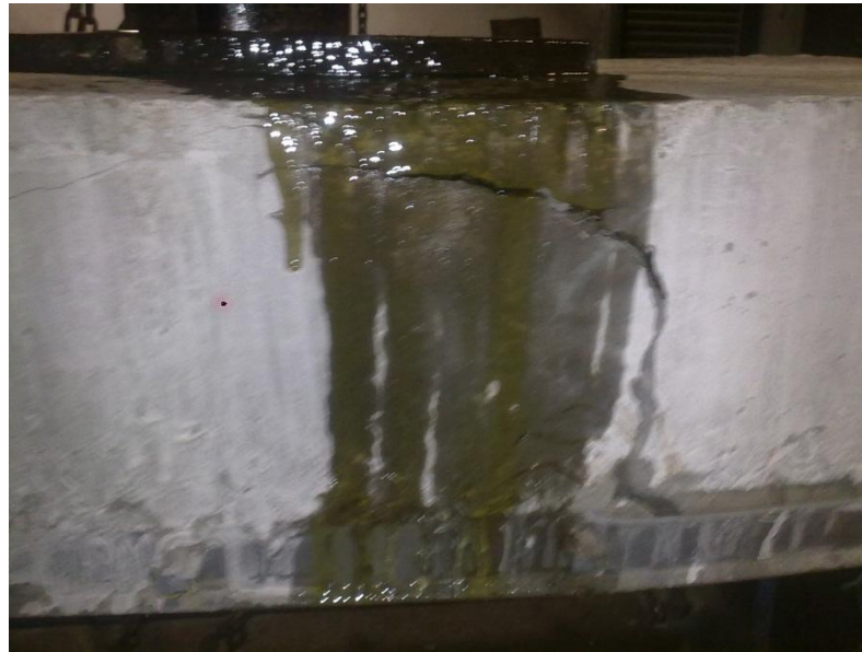
Fig. 6.6 crack in specimen 4
