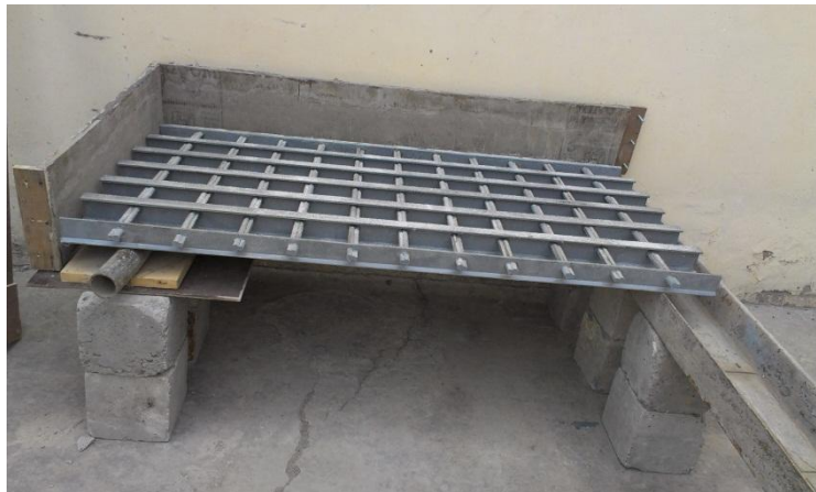
Fig 5.9 setup for casting of beams
