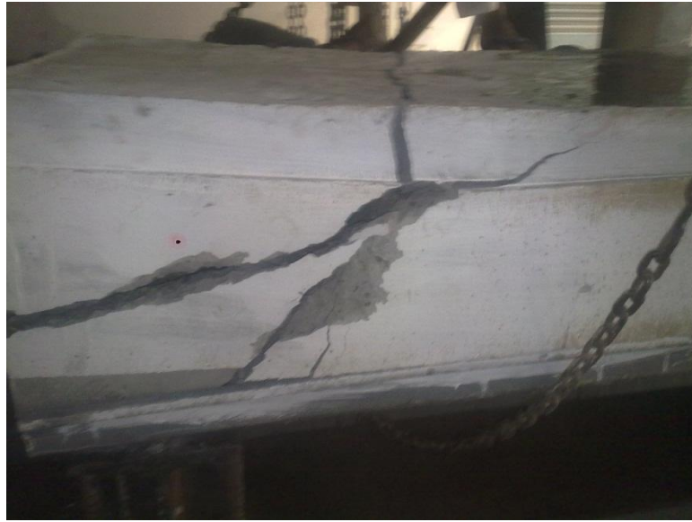
Fig 6.1 flexure shear cracks in specimen 1
