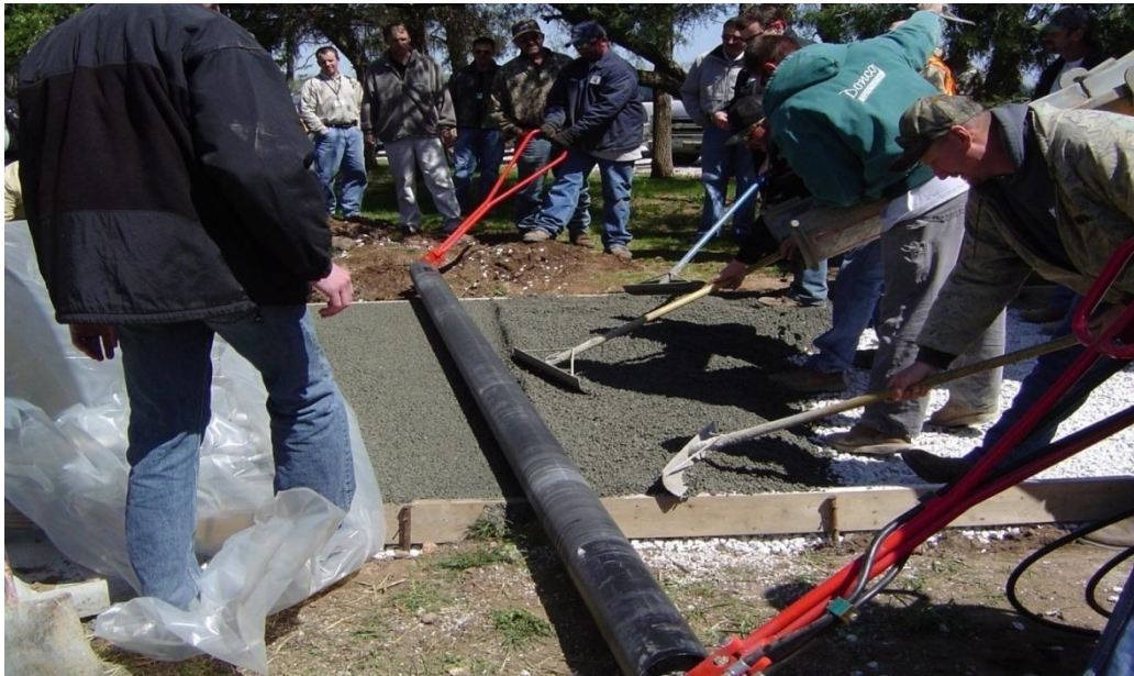
Figure 1.3 Compacting no-fines concrete using roller.
