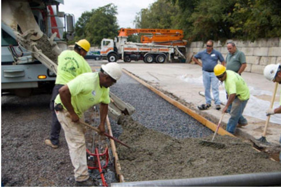
Figure 1.2: Construction Process of no-fines concrete.
