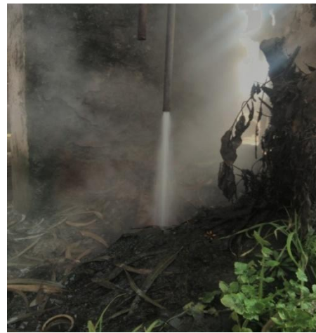
Fig 5.9- drain condensate from steam trap & boiler blow down in industry
