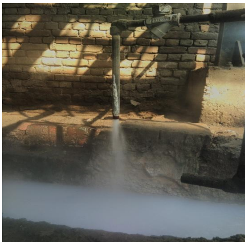
Fig 5.9- drain condensate from steam trap & boiler blow down in industry
