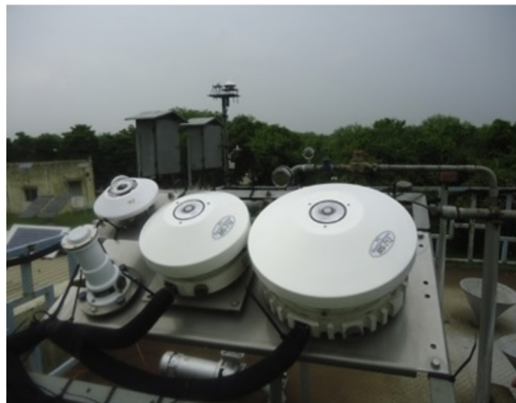
Figure 4.4: Weather Monitoring Station at NISE Gurgaon
