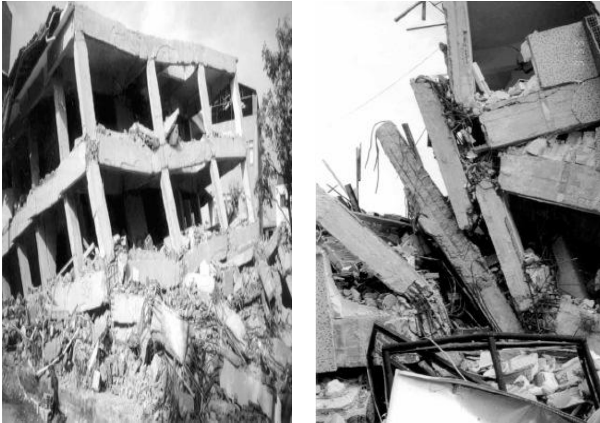
Figure 1.2 Typical beam-column joint failures (1999 Turkey earthquake) [15]
