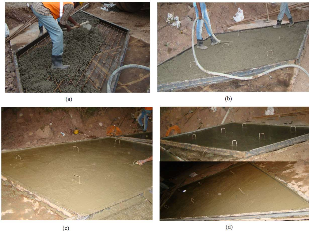
Figure 4.6: Test specimens during concreting S75, S60, S45 and S30: a) pouring concrete in S75 b) Using needle vibrator, c-d) Specimens after concreting
