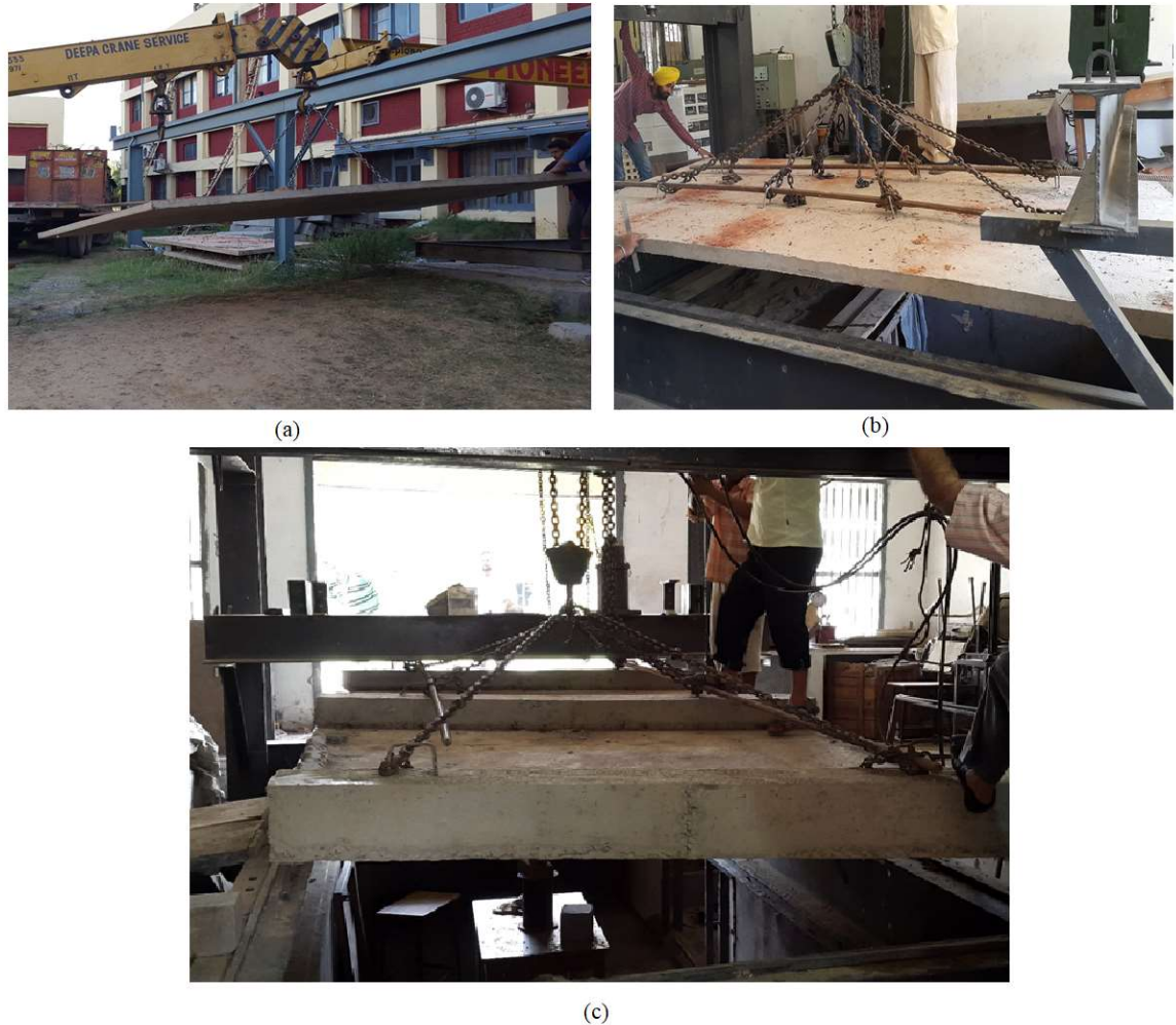
Figure 4.8: Lifting and placing of test specimen on reaction frame- a) lifting from casting yard b-c) Placement of one such specimen non-stiffened and stiffened on reaction frame
