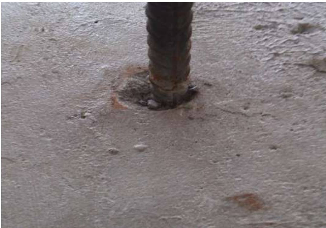
Plate 3.10 Crushing due to pullout bar lugs after pullout test
