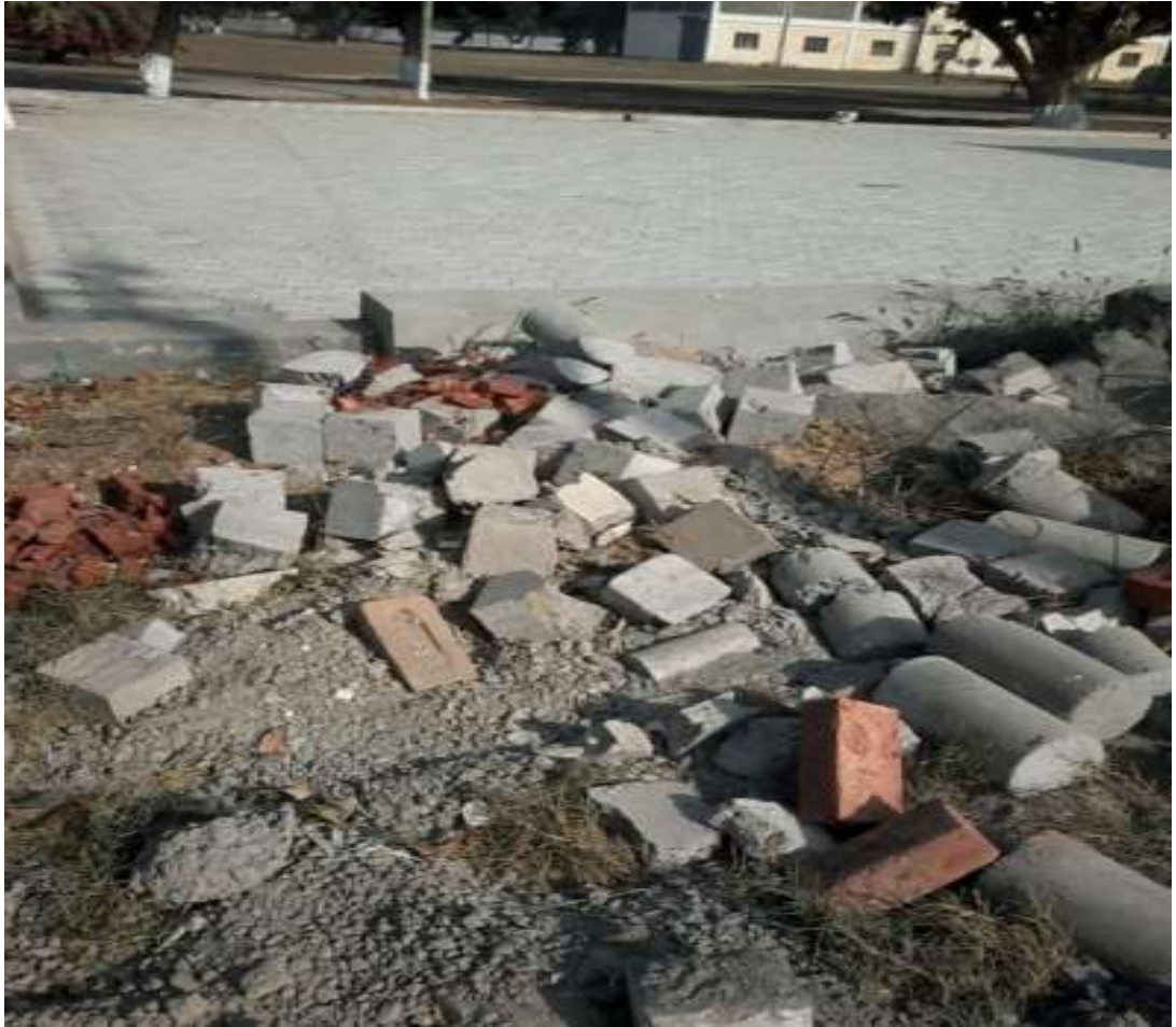
Plate 3.1: Waste concrete rubble used for obtaining RCA
