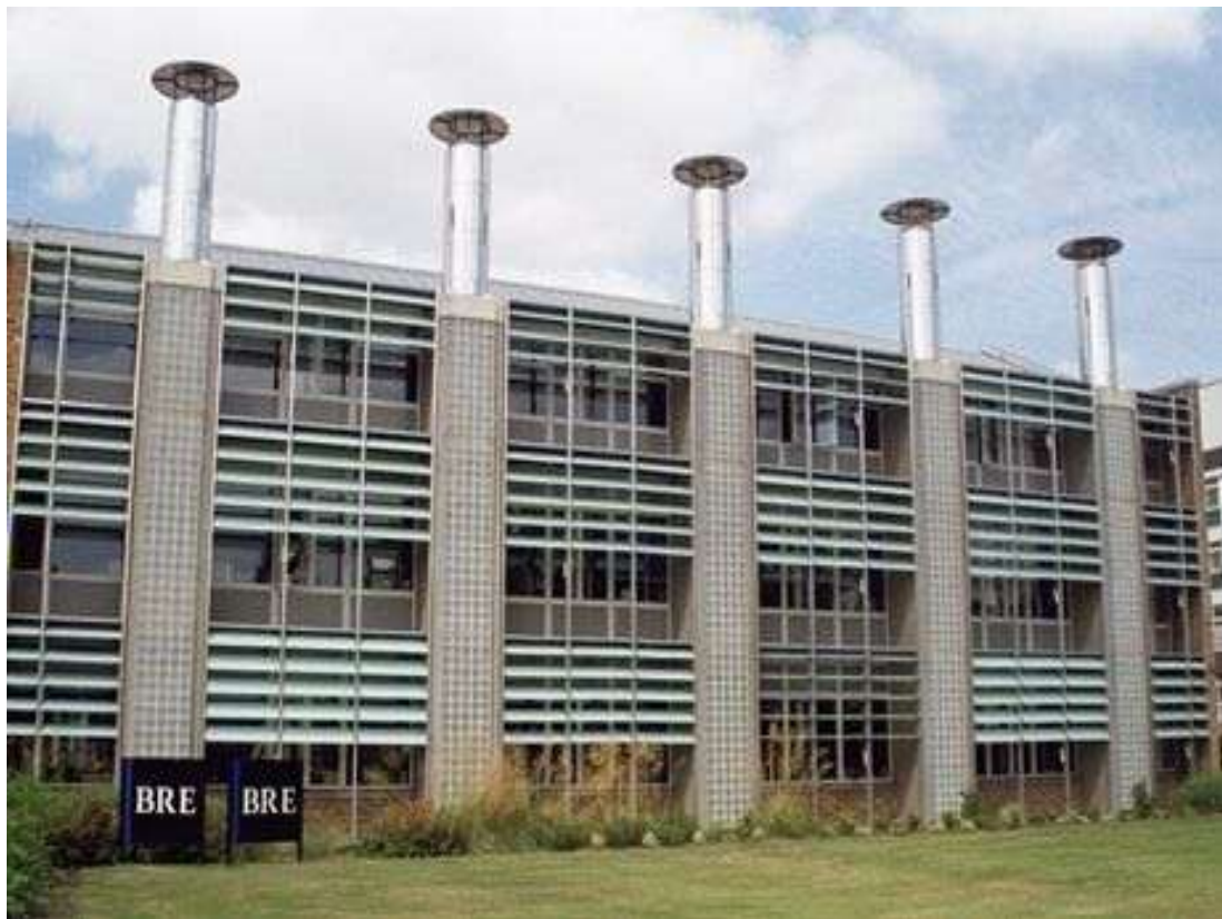
Fig 1.2: The BRE office building ( www.projects.bre.co.uk )
