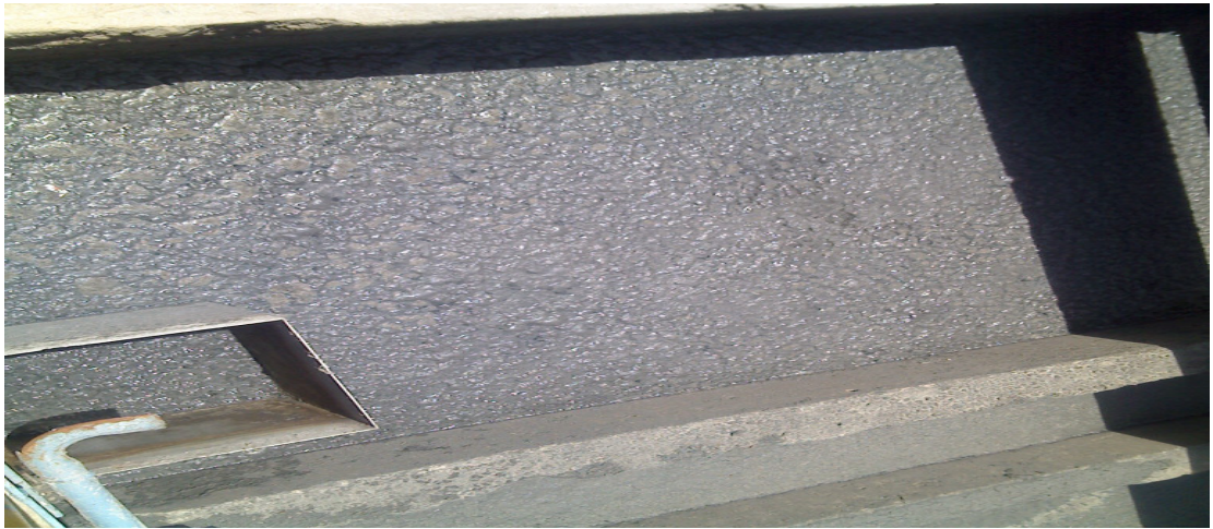
Figure 3.2: Sampling point – Oil and grease trapping unit [P-2]
