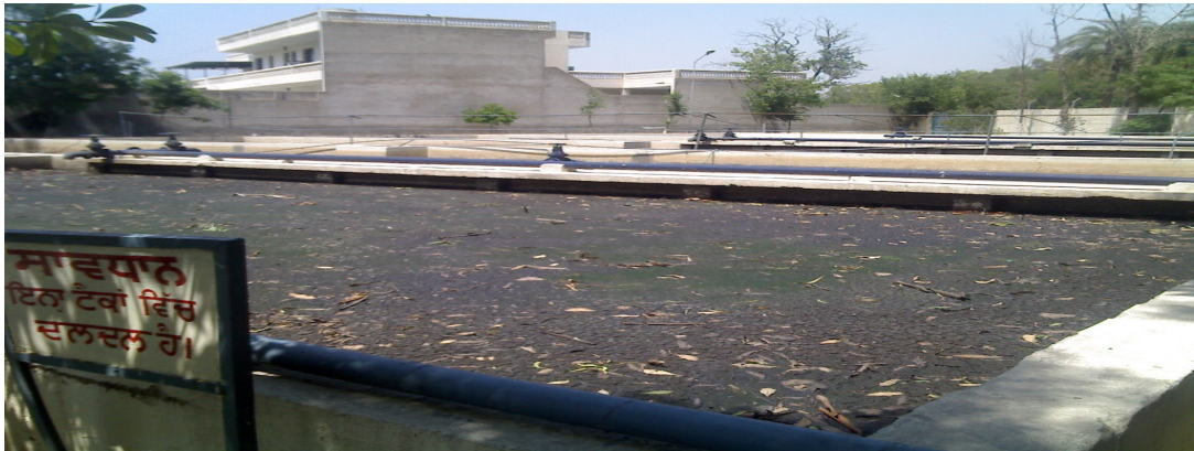
Figure 3.6 Sludge drying beds
