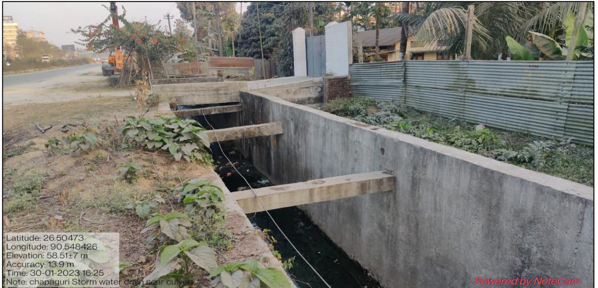
Fig 3.3 storm water drain in chapaguri
