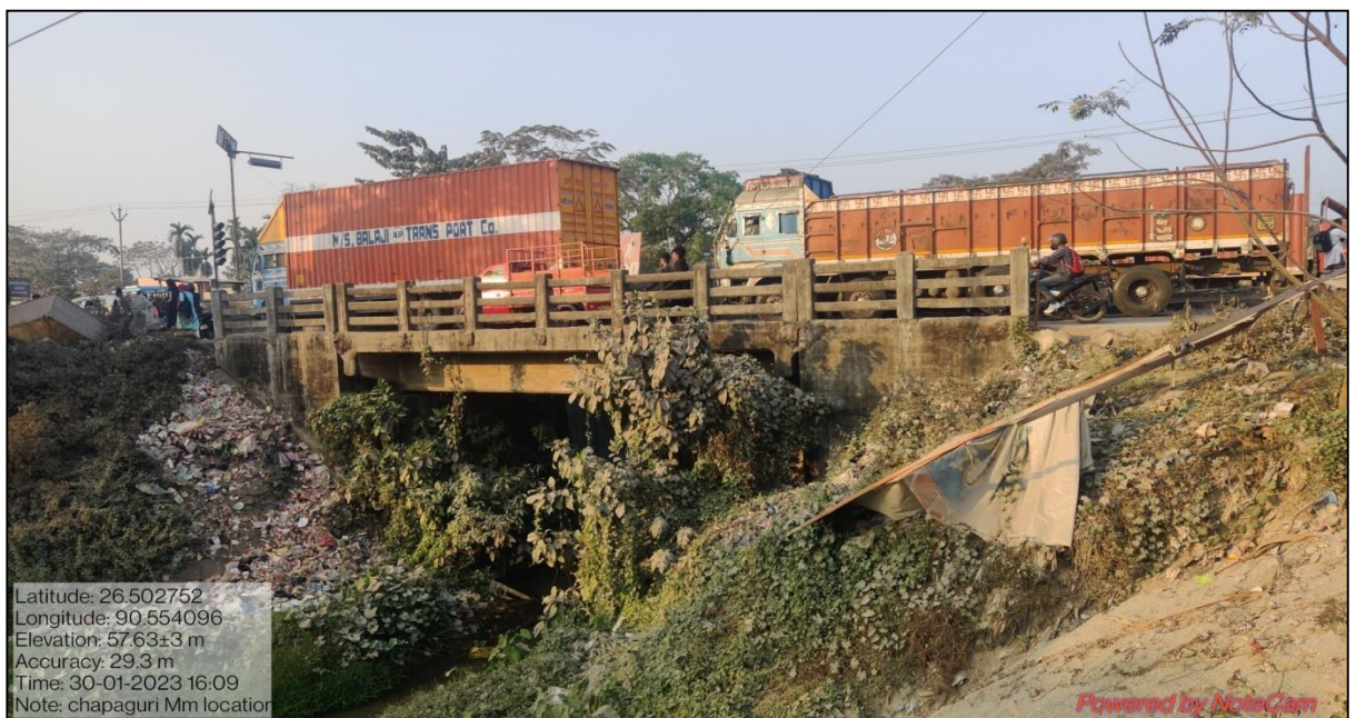
Fig 3.2 Existing minor bridge upon which flyover to be designed
