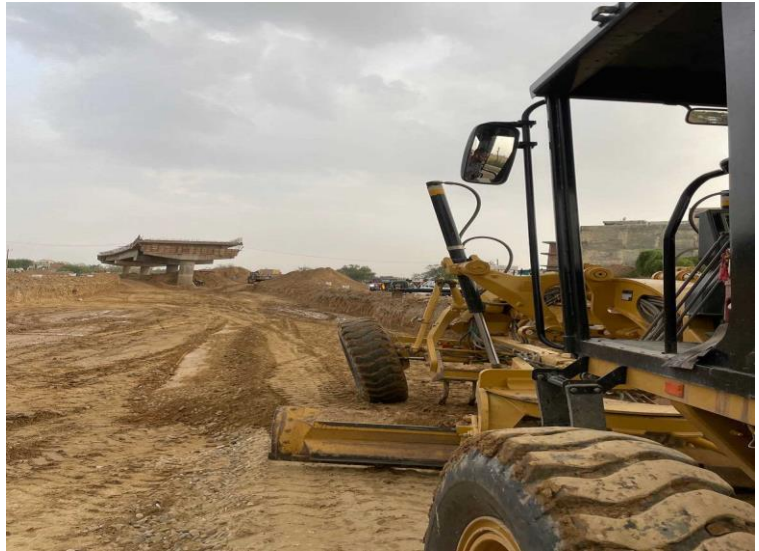
Figure 3.31 (c) Filling of geocell and Spreading of GSB layer
