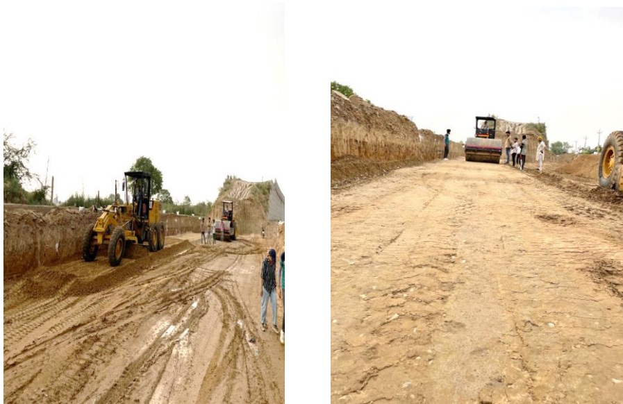
Figure 3.30 Unreinforced Section Instrumentation
