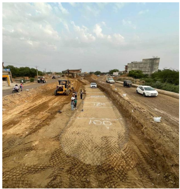
Figure 31(d) Rolling and Compaction of the Surface layer
