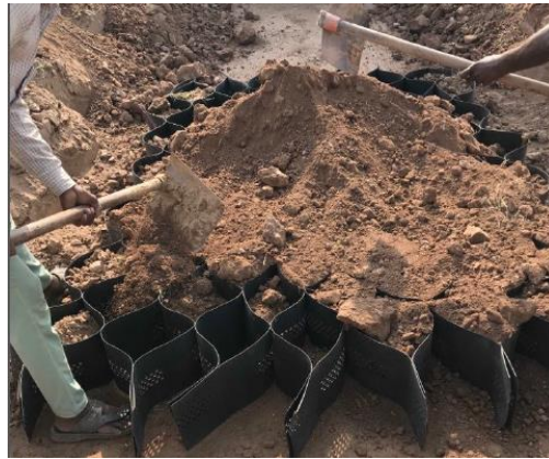
Figure 6.5 Geocell and infill material
