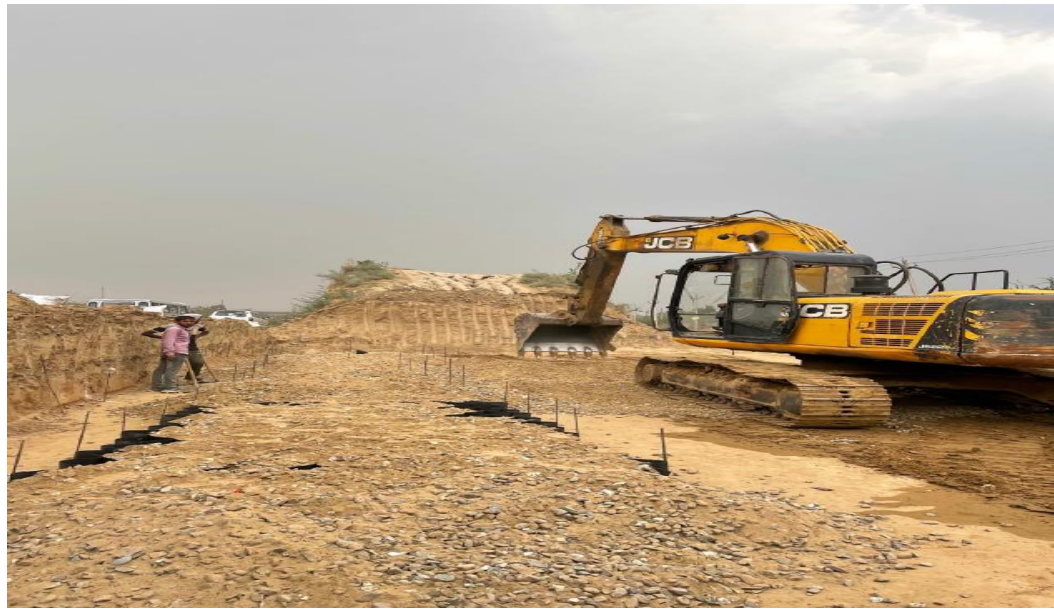
Figure 3.34 Spreading of aggregate materials
