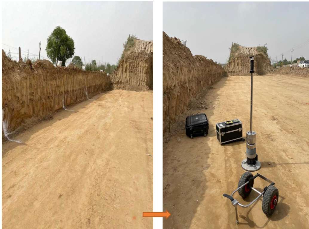
Figure 3.28 Subgrade Preparation on site
