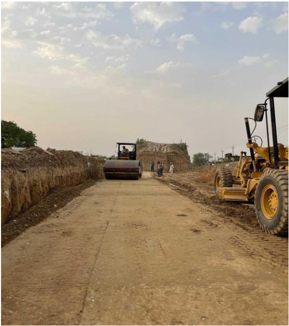
Figure 31(d) Rolling and Compaction of the Surface layer
