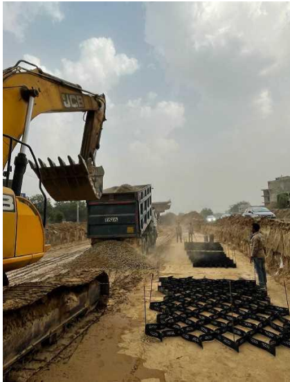
Figure 3.31 (c) Filling of geocell and Spreading of GSB layer
