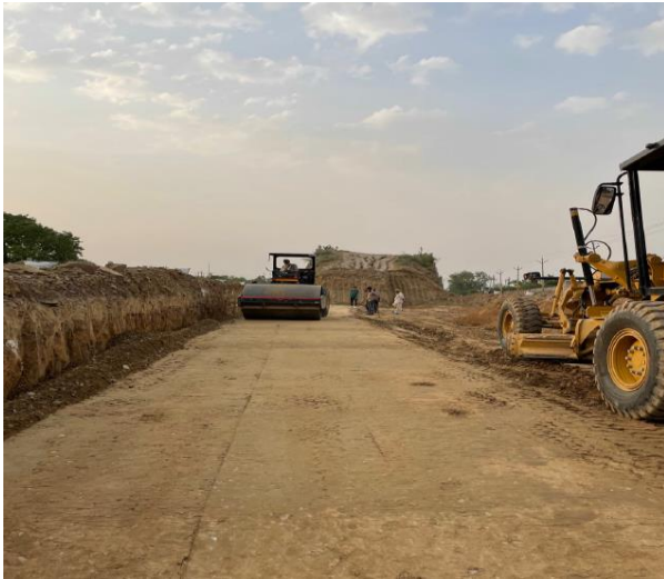
Figure 3.36 Rolling and Compaction of Prepared GSB
