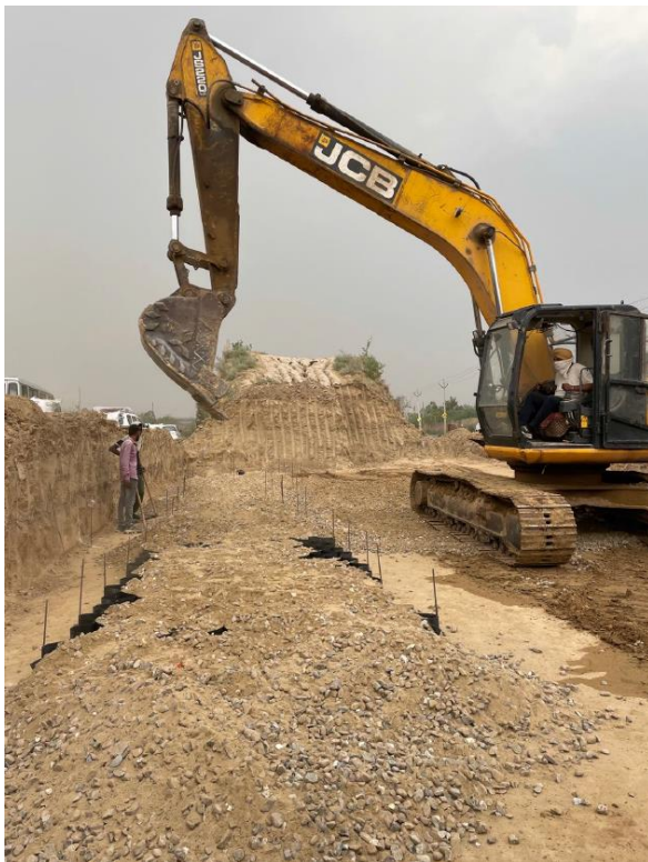
Figure 3.35 Spreading and preparing geocell reinforced sections
