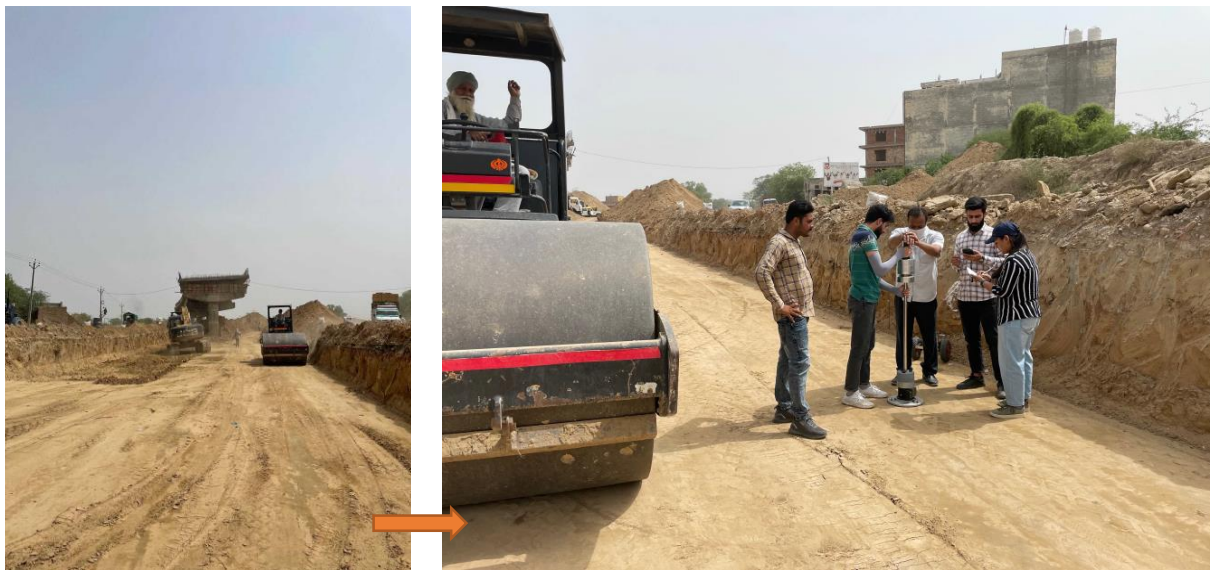
Figure 3.29 LWD Testing on prepared Subgrade
