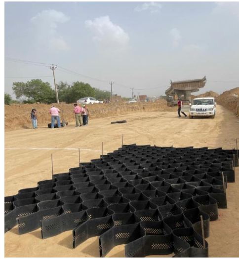
Figure 31(a) Laying of Geocell
