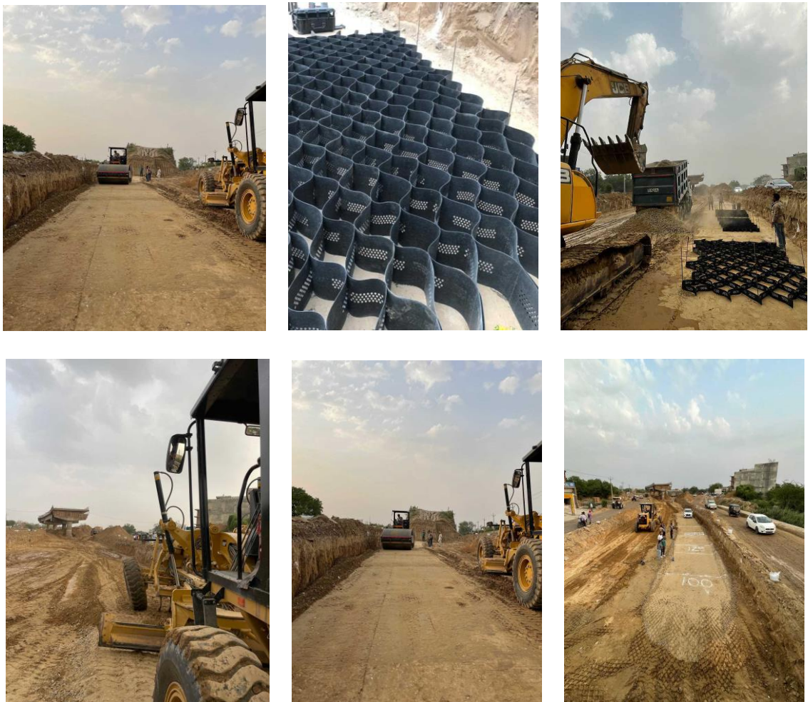
Fig 2.2 Various stages of laying Geocell
