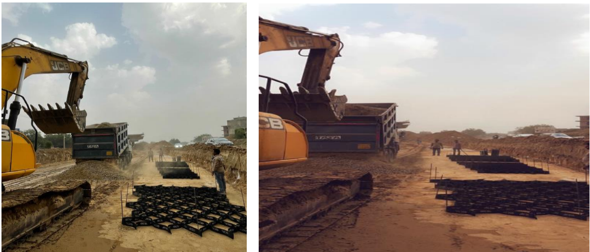
Figure 3.33 Filling of Geocells
