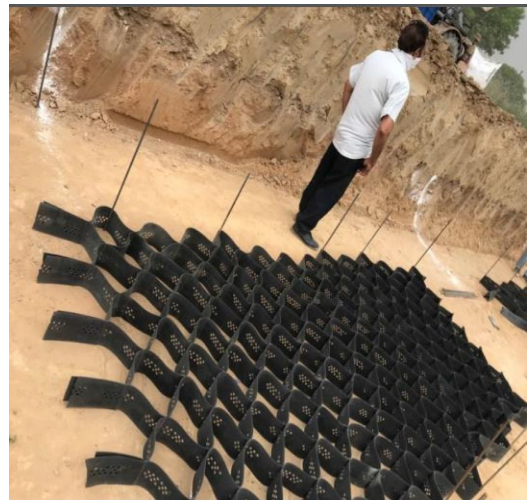
Figure 31(b) Spreading and Anchoring of Geocell
