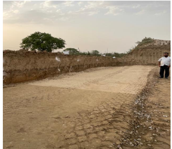
Figure 3.36 Rolling and Compaction of Prepared GSB
