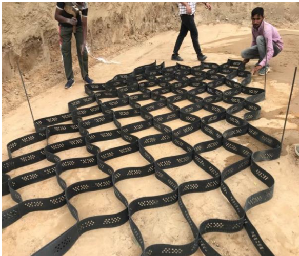
Figure 31(b) Spreading and Anchoring of Geocell
