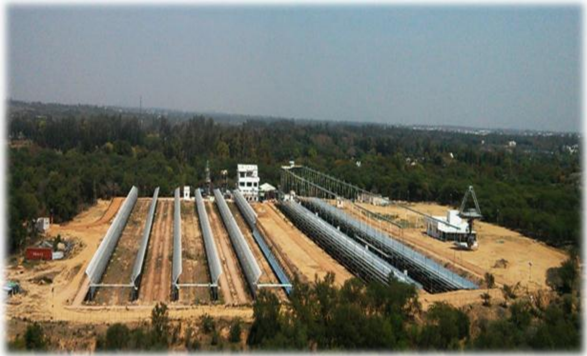
Figure 3.1 Test facility of 1 MW CSP plant employing PTC and LFR solar fields, [NISE, India]
