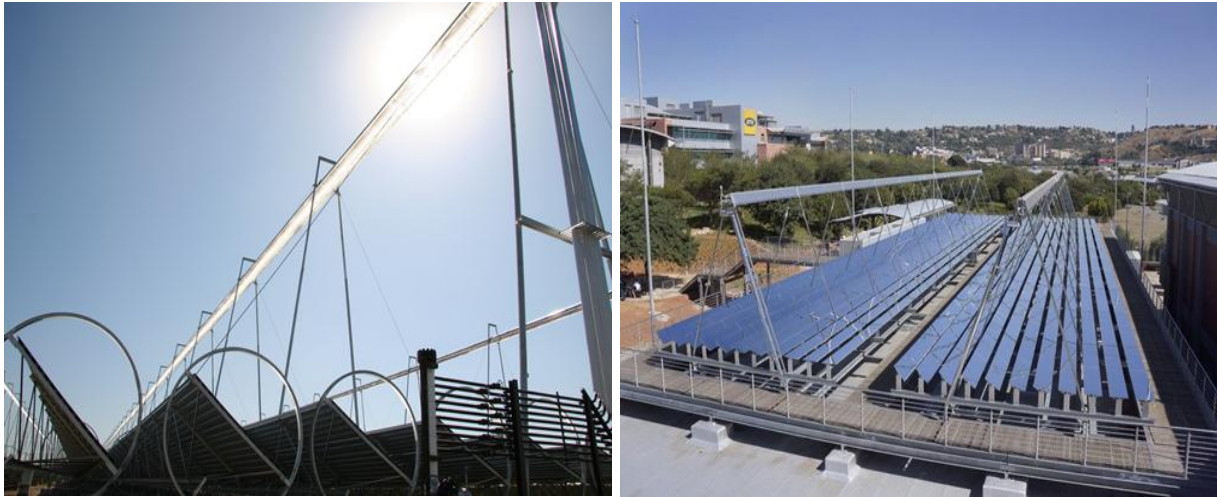
Figure 2.8 Linear fresnel reflector [Mills et al., 2000]
