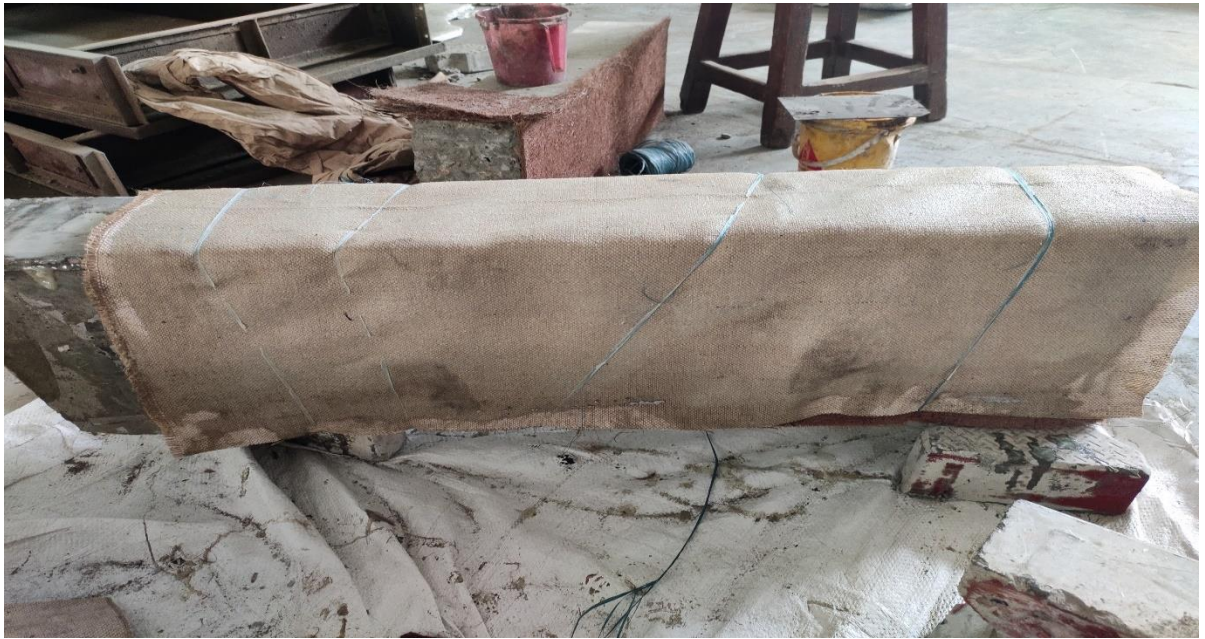
Figure 3.5 – Beam after U-Type retrofitting using flax fiber
